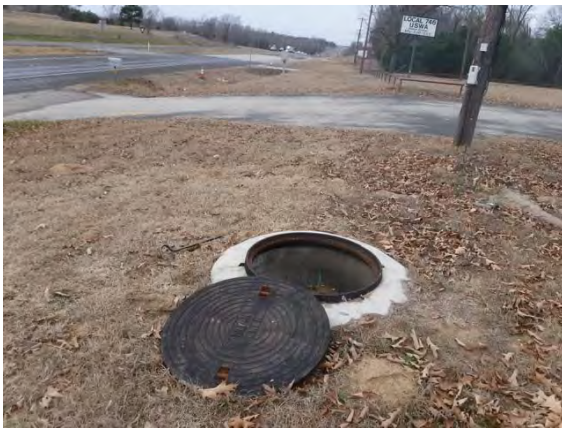
ARV 2050 Highway 31 West Manhole and Area in Good Condition
