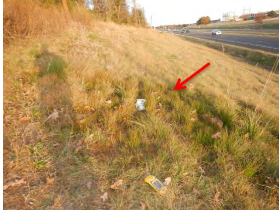
Highway 31 West Wet Spot 243' East of 13838; Leak to needing to be identified
