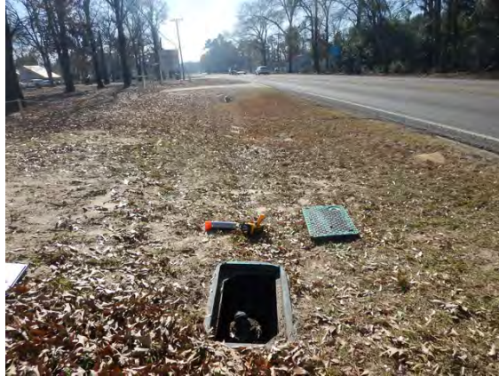
ARV 1260 Pilot Area and Vault in Good Condition
