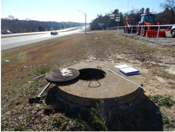
ARV 1310 Rustic Area and Manhole in Good Condition
