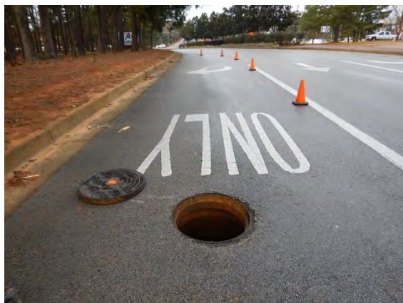
ARV 1300 Crossing Manhole Ring and Cover in Good Condition
