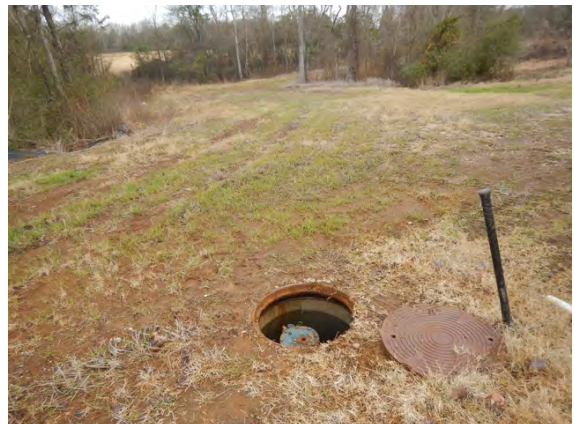
ARV 1231 Shackleford Manhole and Area in Good Condition
