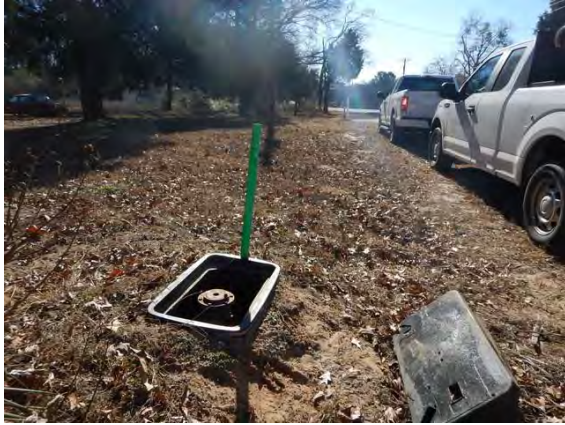
ARV 1291 Pilot Area and Vault in Good Condition
