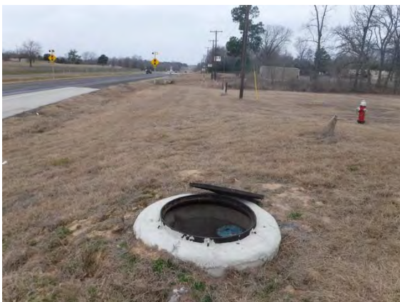
ARV 2060 Highway 31 West Area and Manhole in Good Condition
