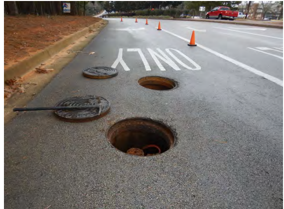
ARV 1230 Shackleford Manhole and Area in Good Condition
