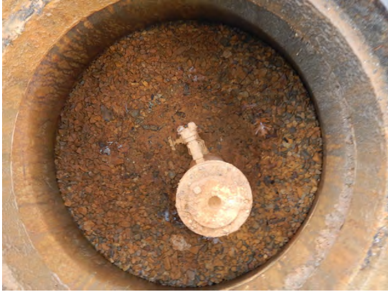
ARV 2020 East Grande Air Release Valve in Good Condition; Force Main not Visible
