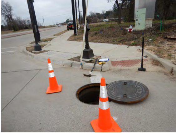
ARV 1330 Oak Creek Area and Manhole in Good Condition
