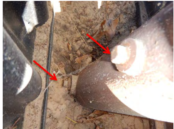
ARV 1291 Pilot Arv Body with Capped Valve Locations
