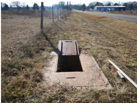
ARV 1271 Pilot Area and Vault in Good Condition
