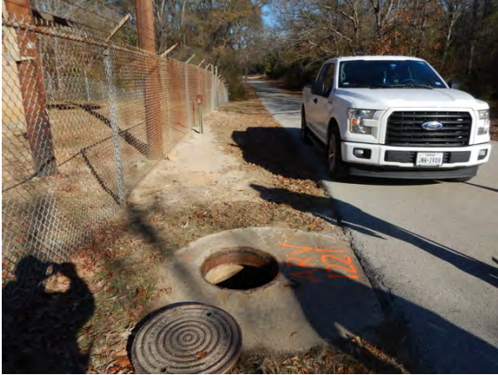
ARV 1221 Bellwood Manhole and Area in Good Condition
