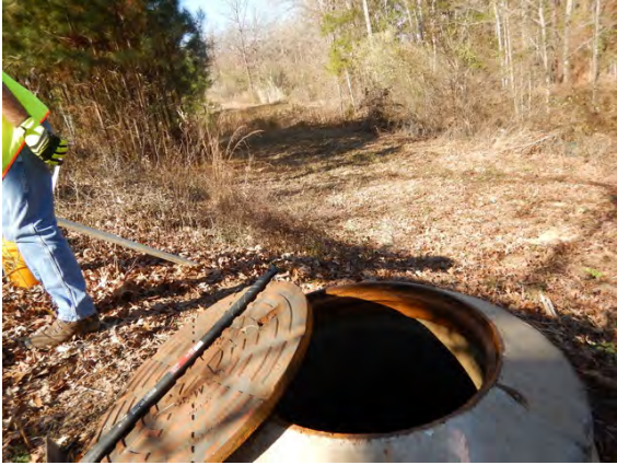
ARV 1350 Nottingham Area and Manhole in Good Condition
