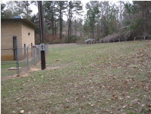
Sloping Ground Adjacent to Westside of Building
