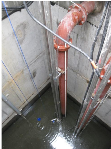
Wet Well Interior
