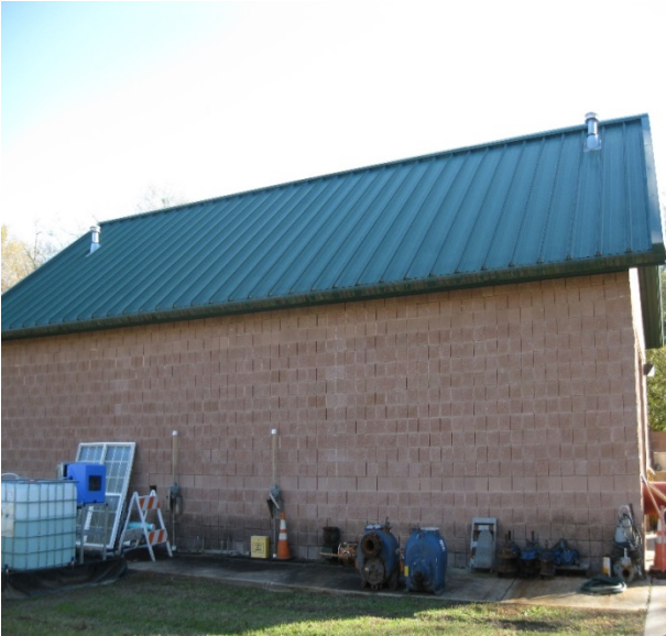
Lift Station Building Facing West
