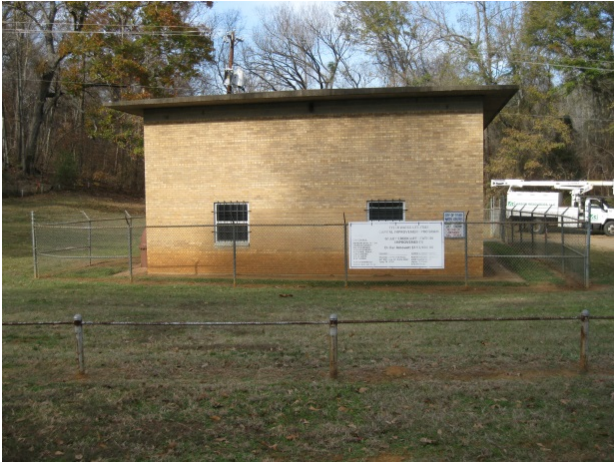
Lift Station Perimeter Facing South
