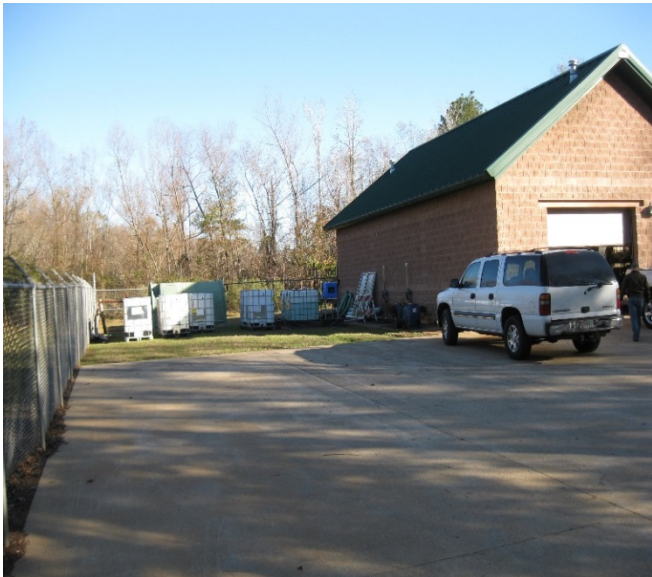
Lift Station Perimeter To Left of Building Facing North
