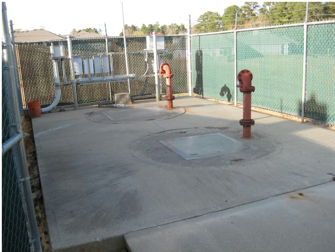
Lift Station Perimeter
