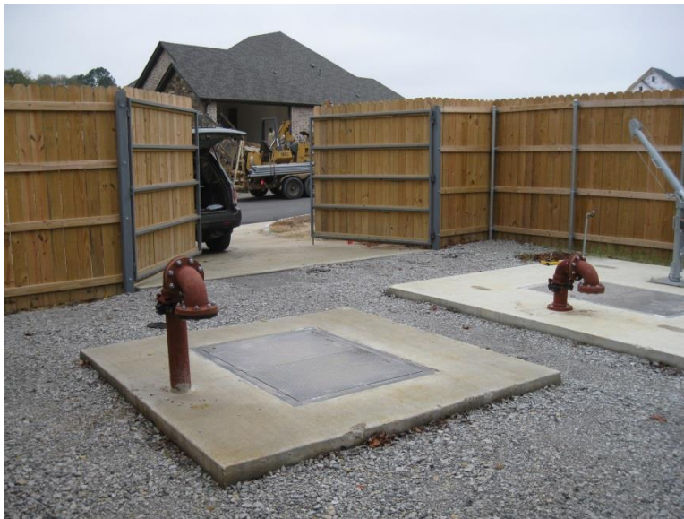
Life Station Gate and Wet Well and Valve Vault Slabs
