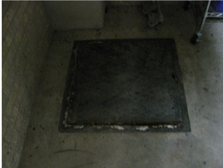
Hatch Could Not Be Opened Without Tools
