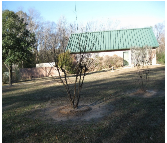
Lift Station Building Facing East
