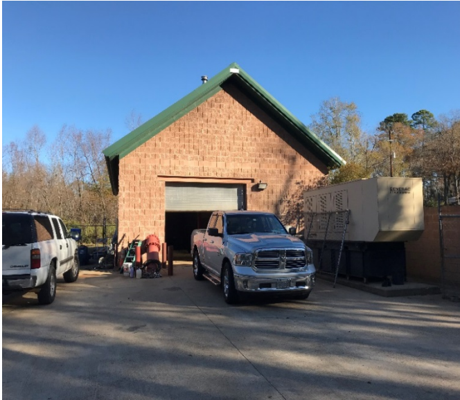
CMU Lift Station Building Facing North
