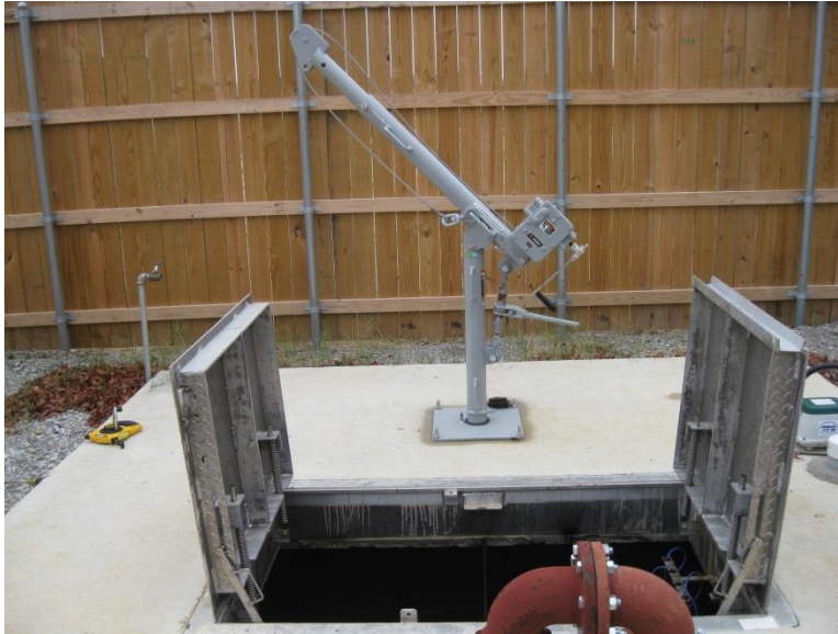
Crane Near Wet Well
