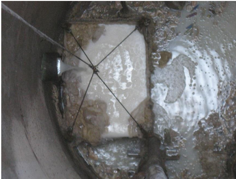
Wet Well Interior
