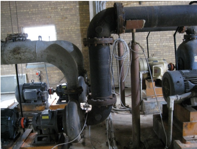
Cornell and Gorman - Rupp Pumps in Series (3 sets of 2 pumps each)
