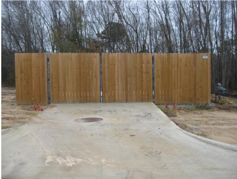
Lift Station Perimeter Fence
