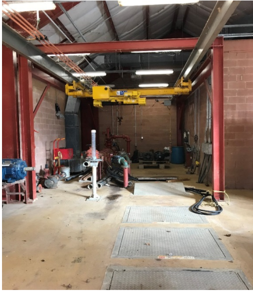
Interior of Building Facing North
