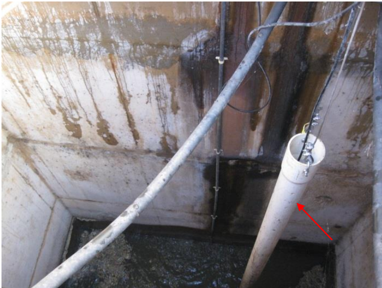
Interior of Wet Well
