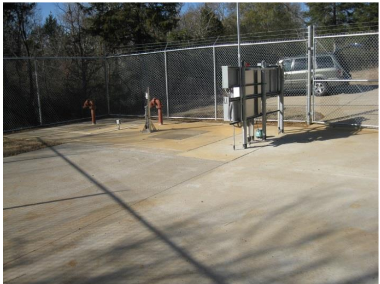
Wet Well Slab Surface Flush With Ground
