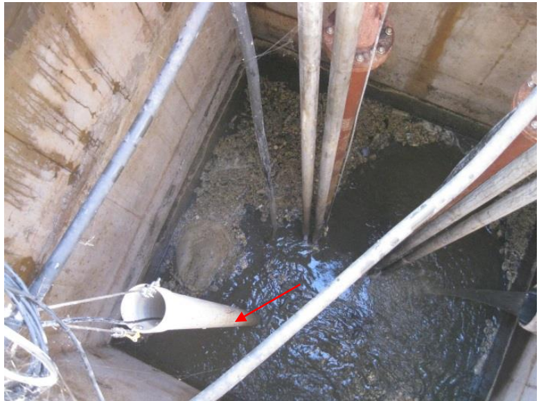
Interior of Wet Well (2)
