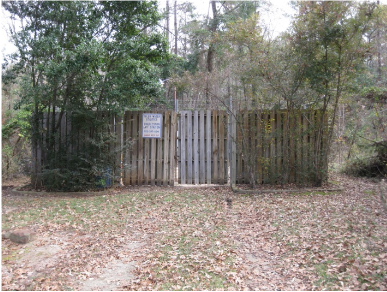
Lift Station Perimeter Facing North
