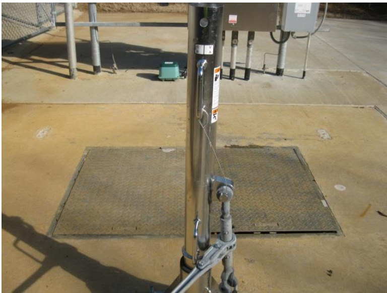
Wet Well Slab
