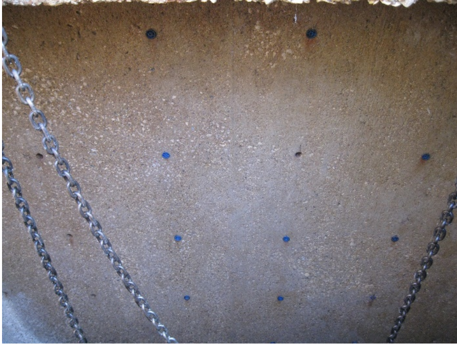
Wet Well Walls in Good Condition
