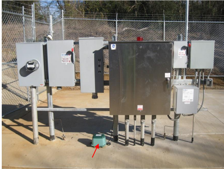
Air Compressor For Aeration of Wet Well
