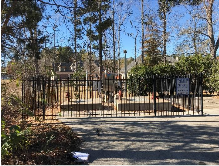
Lift Station Perimeter Facing West
