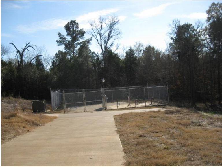
Lift Station Perimeter
