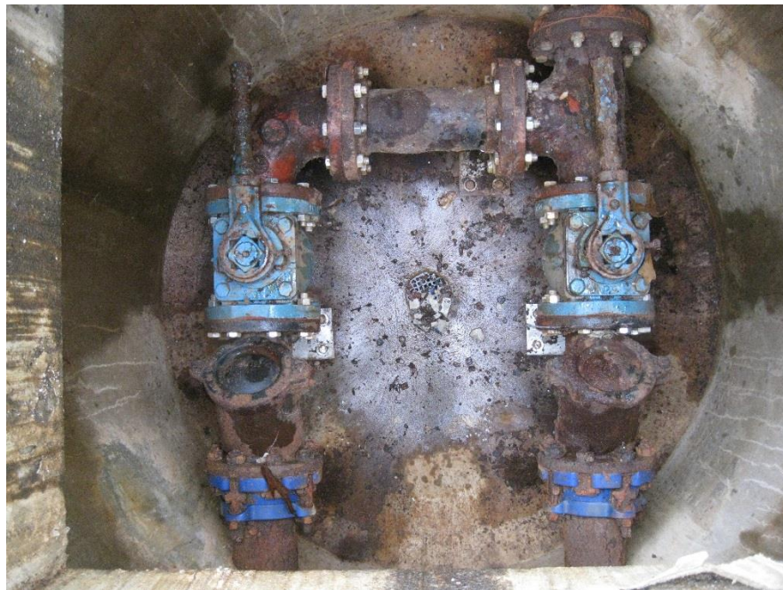
Valve Vault Interior
