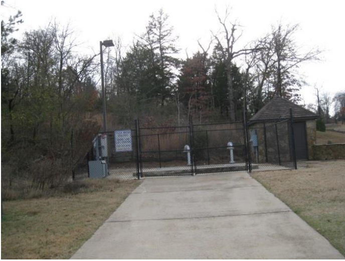
Lift Station Perimeter Facing South
