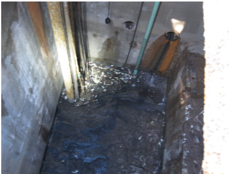
Wet Well Concrete Walls in Good Condition
