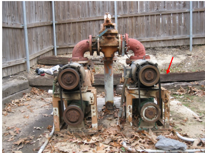
Ground From North Side Sloped Towards Wet Well Slab. Railroad Tie Retaining Wall Visible Behind Pumps
