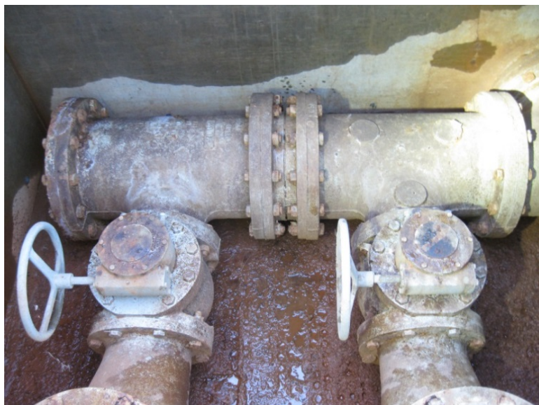
Valve Vault Interior
