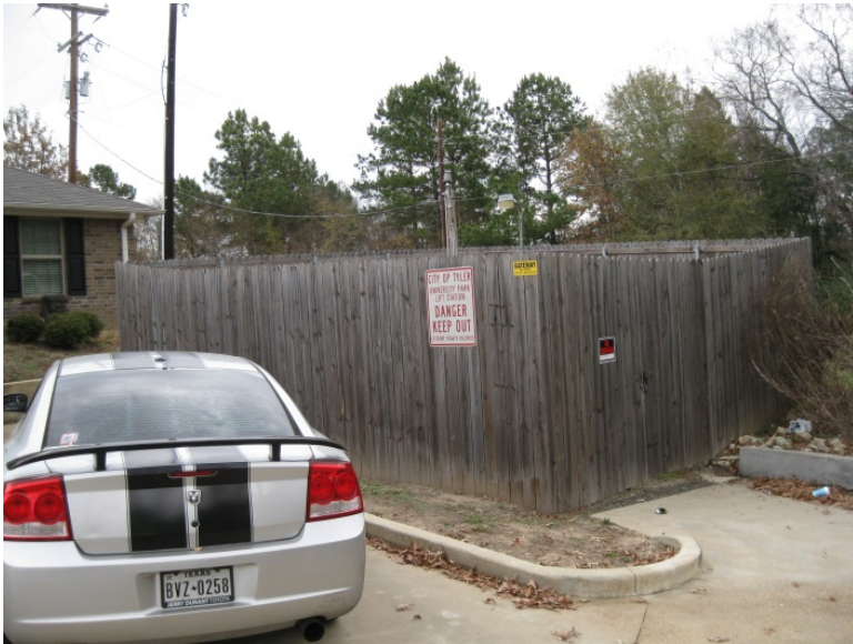
Lift Station Perimeter Facing North
