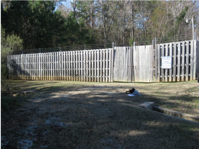
Lift Station Perimeter Facing West
