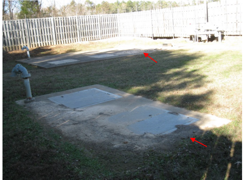
Valve Vault and Wet Well Slab Flush With Natural Ground
