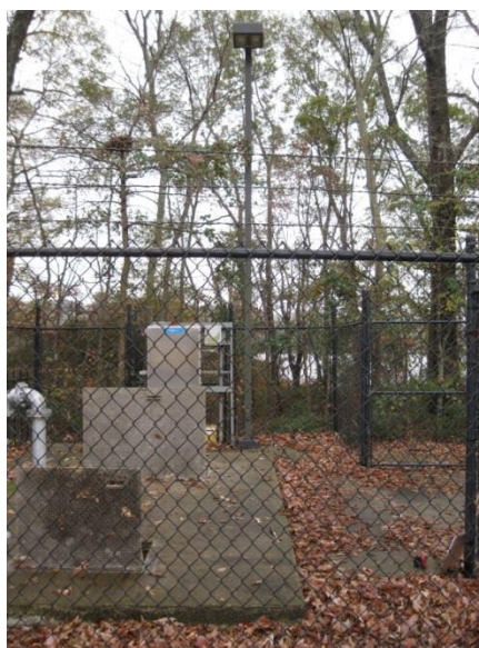
Lift Station Wet Well Slab
