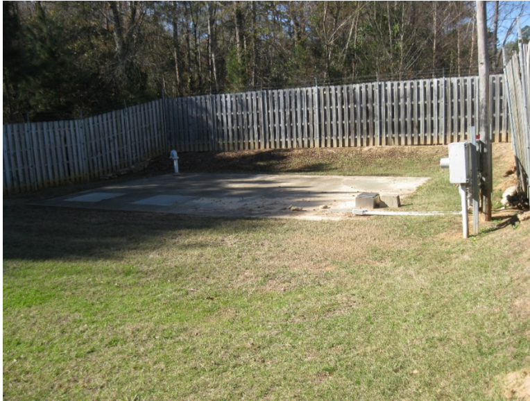
Lift Station Perimeter Facing East
