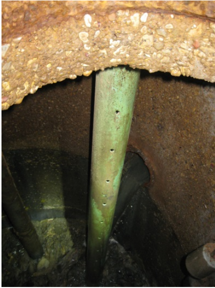
Wet Well Interior
