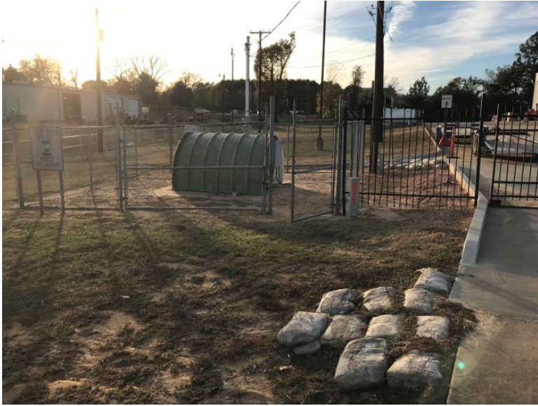
Lift Station Perimeter Facing West
