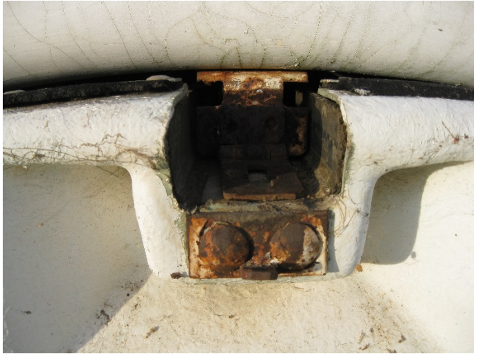
Lift Station Dog House Rear- Facing East
