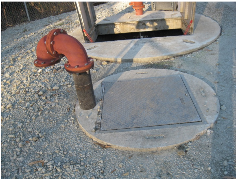
Exterior of Valve Vault and Vent Pipe
