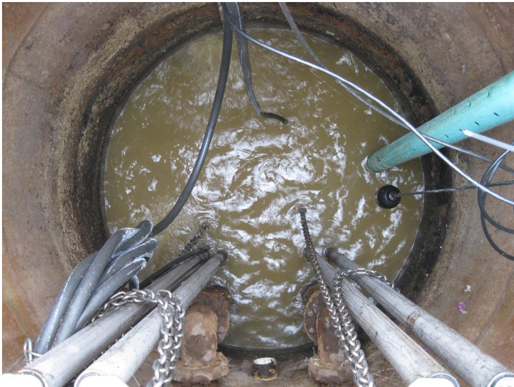
Wet Well in Good Condition
