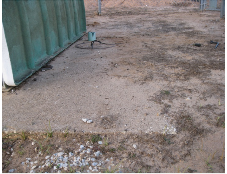
Lift Station Perimeter Facing West
