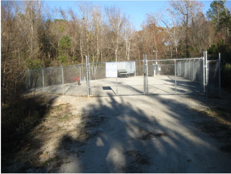
Lift Station Perimeter Facing West
