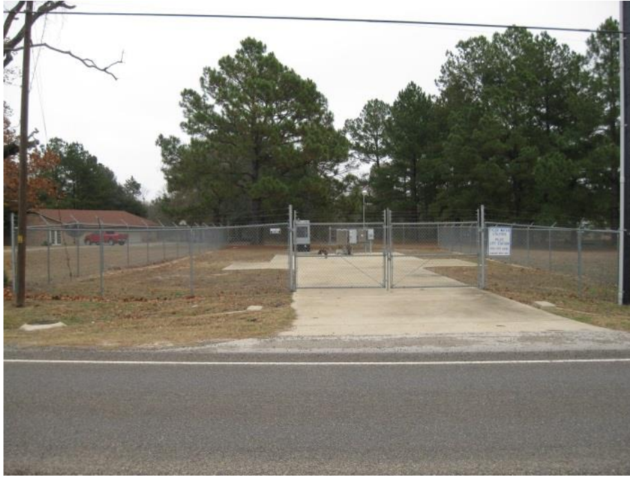
Lift Station Perimeter Facing East
