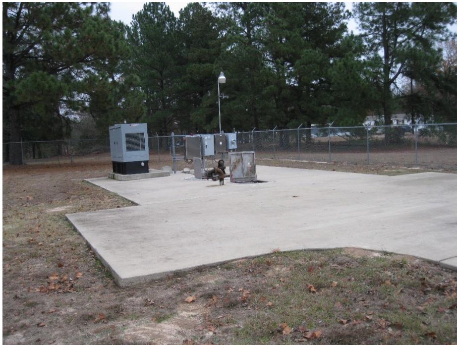
Lift Station Grounds Facing Southeast
