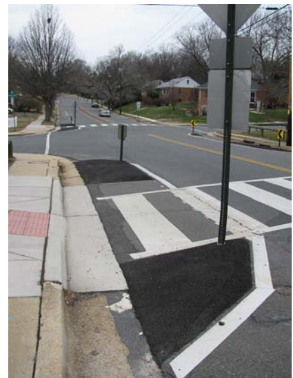
Figure B-17: Simple Curb Extension
