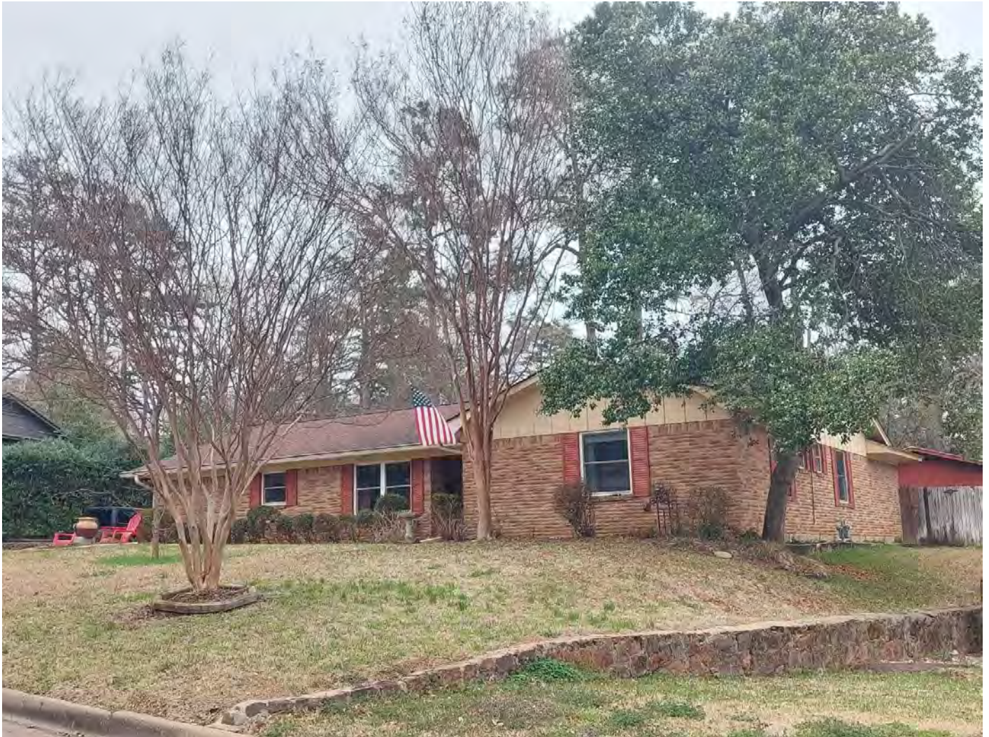
Photo 2. Retaining wall in the 2900 block of Pollard Drive. Camera facing southwest.
