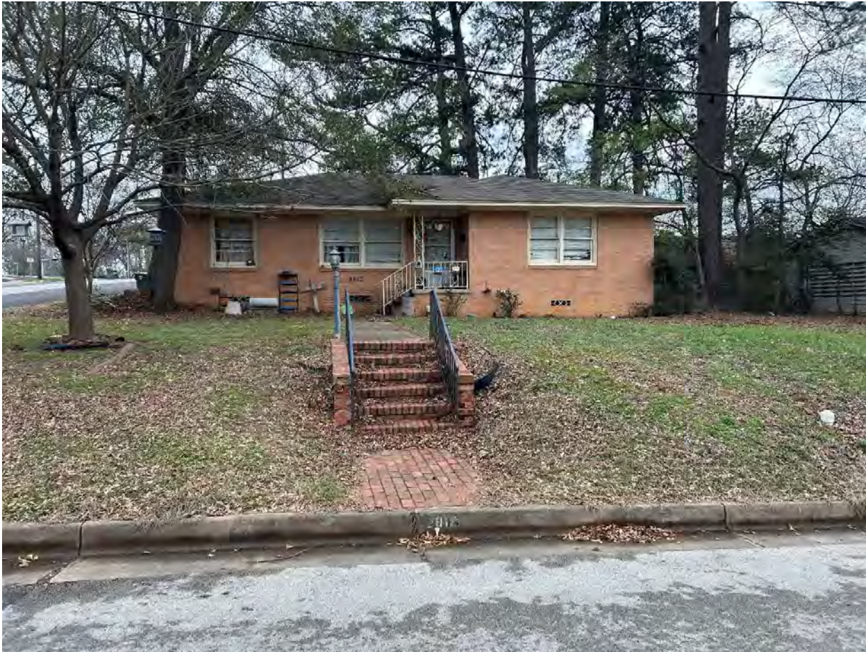
Photo 24. Front façade of 2812 Dinah Lane (Resource 139678). Camera facing east.
