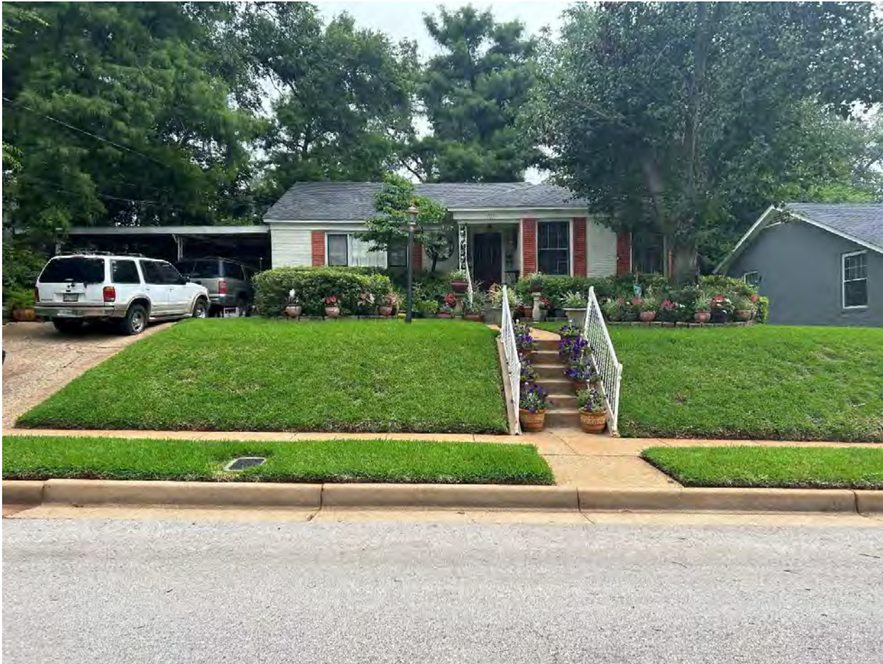
Photo 22. Front façade of 702 E. Hudson Street (Resource 139883). Camera facing north.
