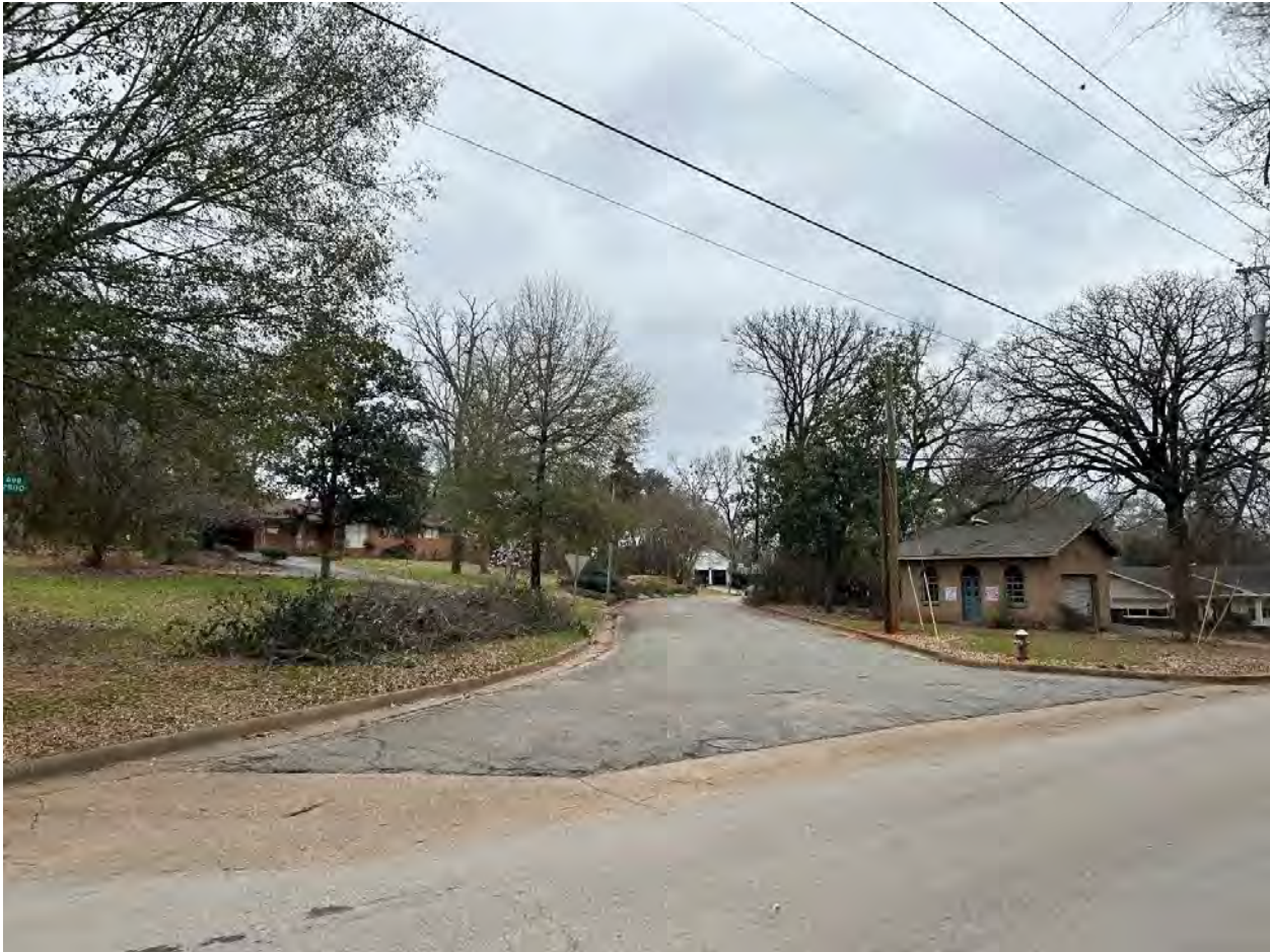
Photo 17. Contextual view of the pump house at 2917 Jan Avenue (Resource 136297). Camera facing southwest.
