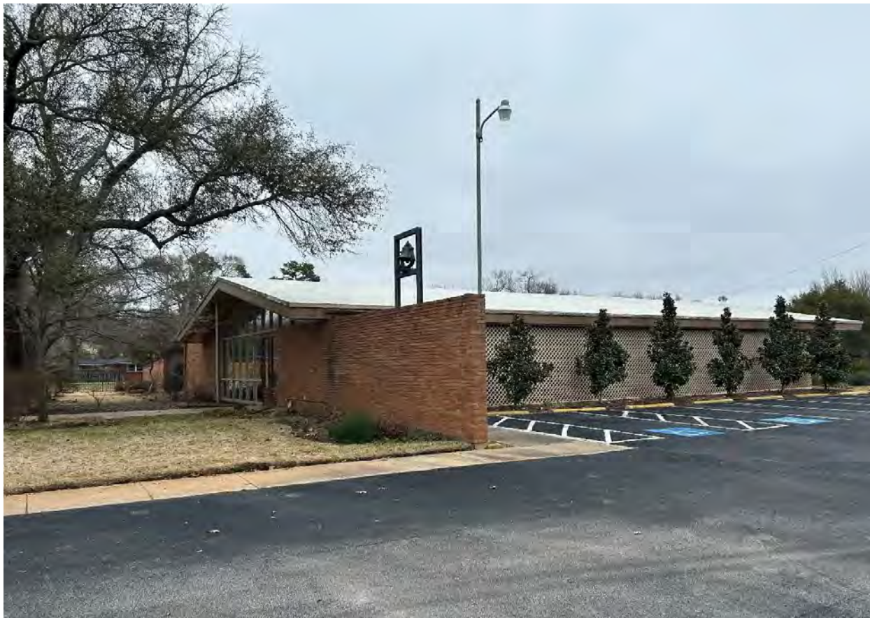
Photo 15. Oblique of St. Francis Episcopal Church at 3232 Jan Avenue A (Resource 136374). Camera facing northeast.
