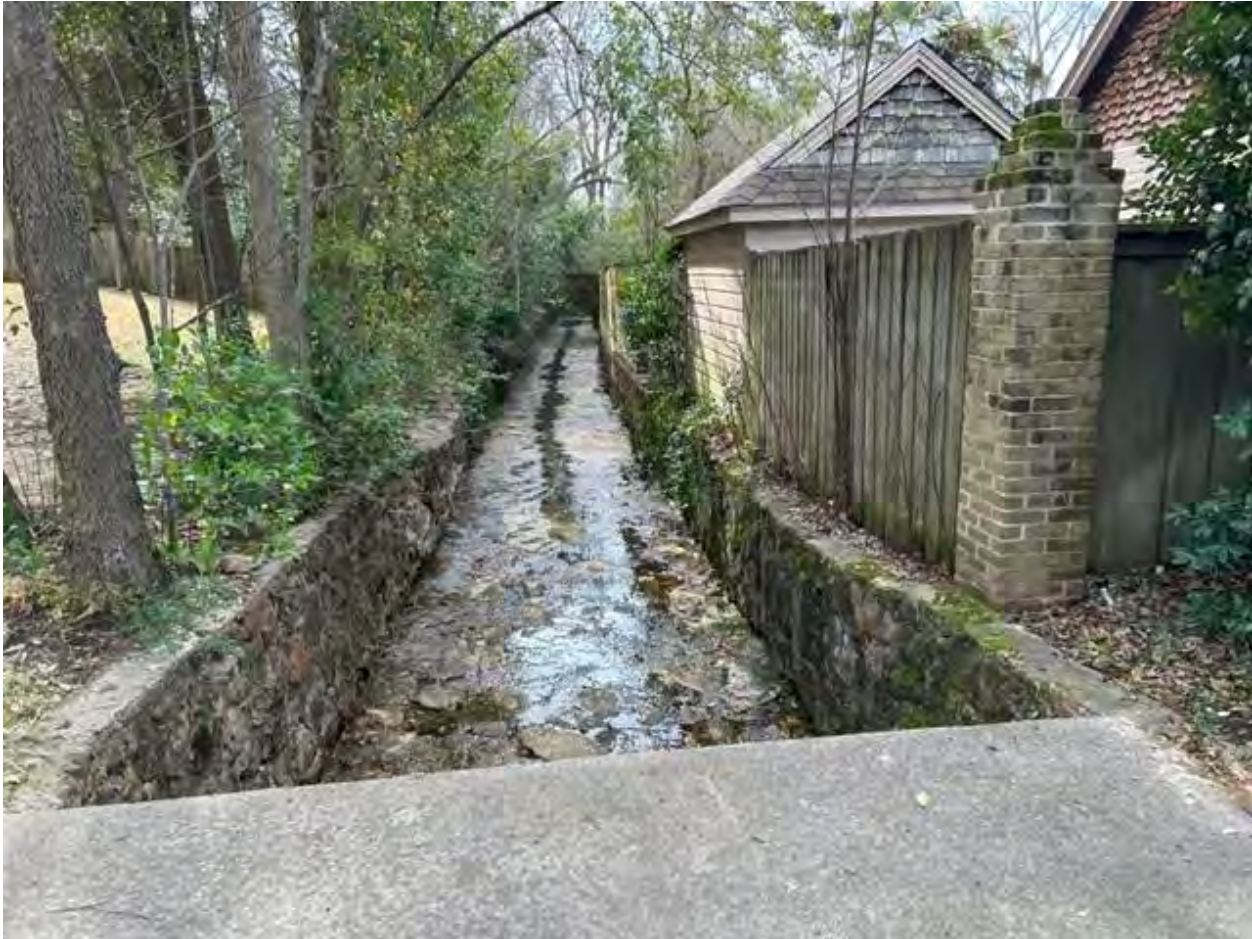
Photo 20. Stone-lined drainage (Resource 139655) near 1005 E. Amherst Street. Camera facing south.
