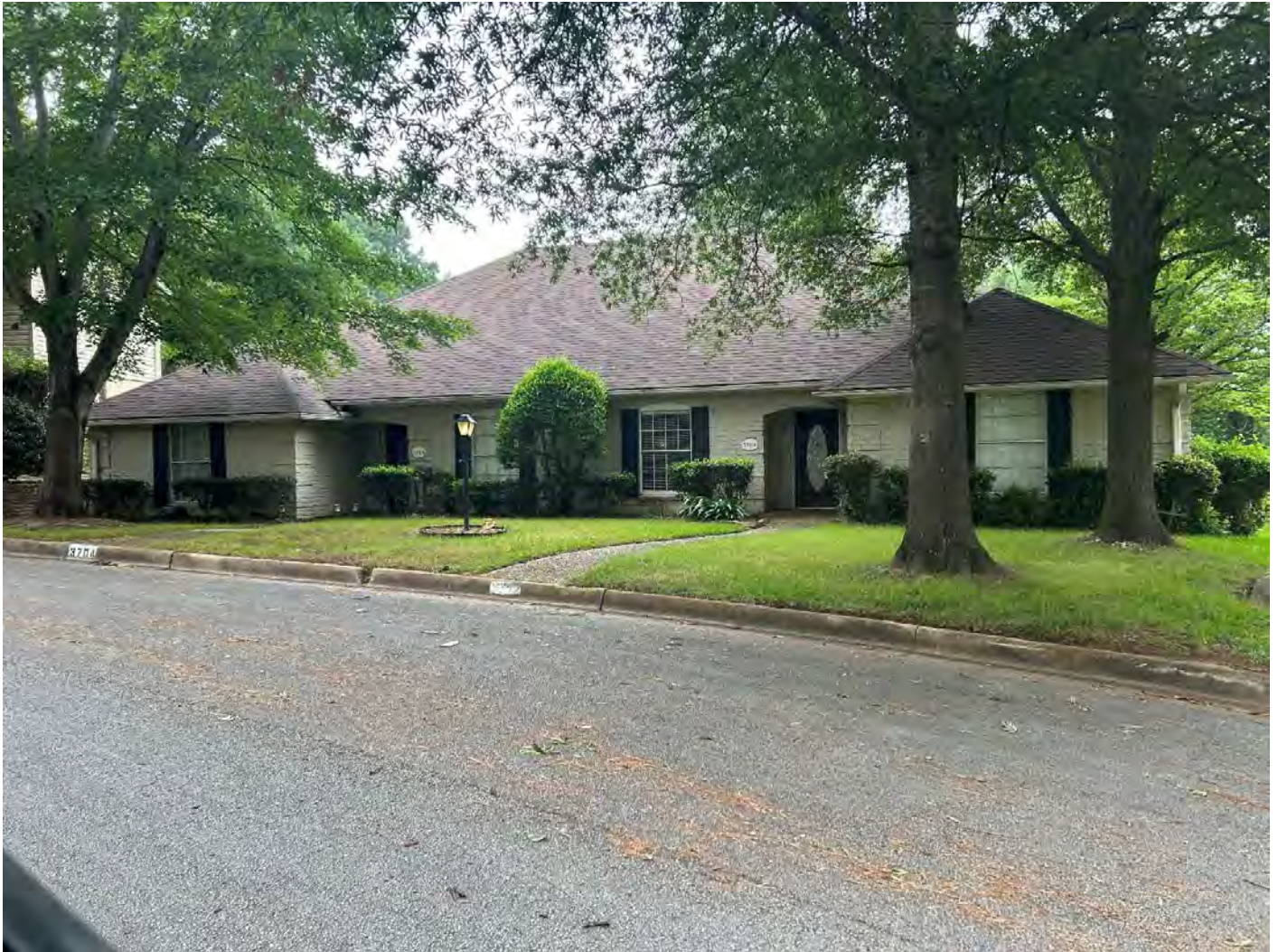
Photo 6. Oblique view of a duplex at 3704 Colony Park Drive (Resource 139787). Camera facing south.
