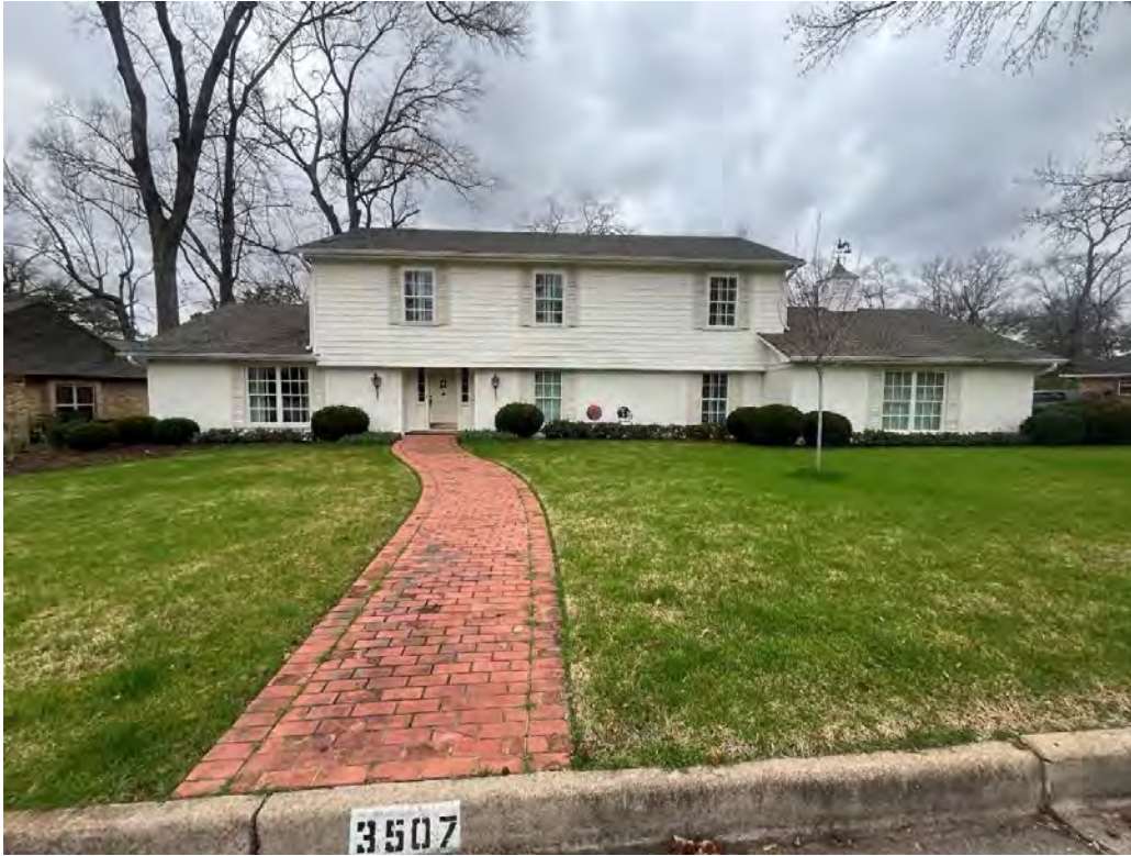
Photo 37. Front façade of 3507 Fry Avenue (Resource 138173). Camera facing west.
