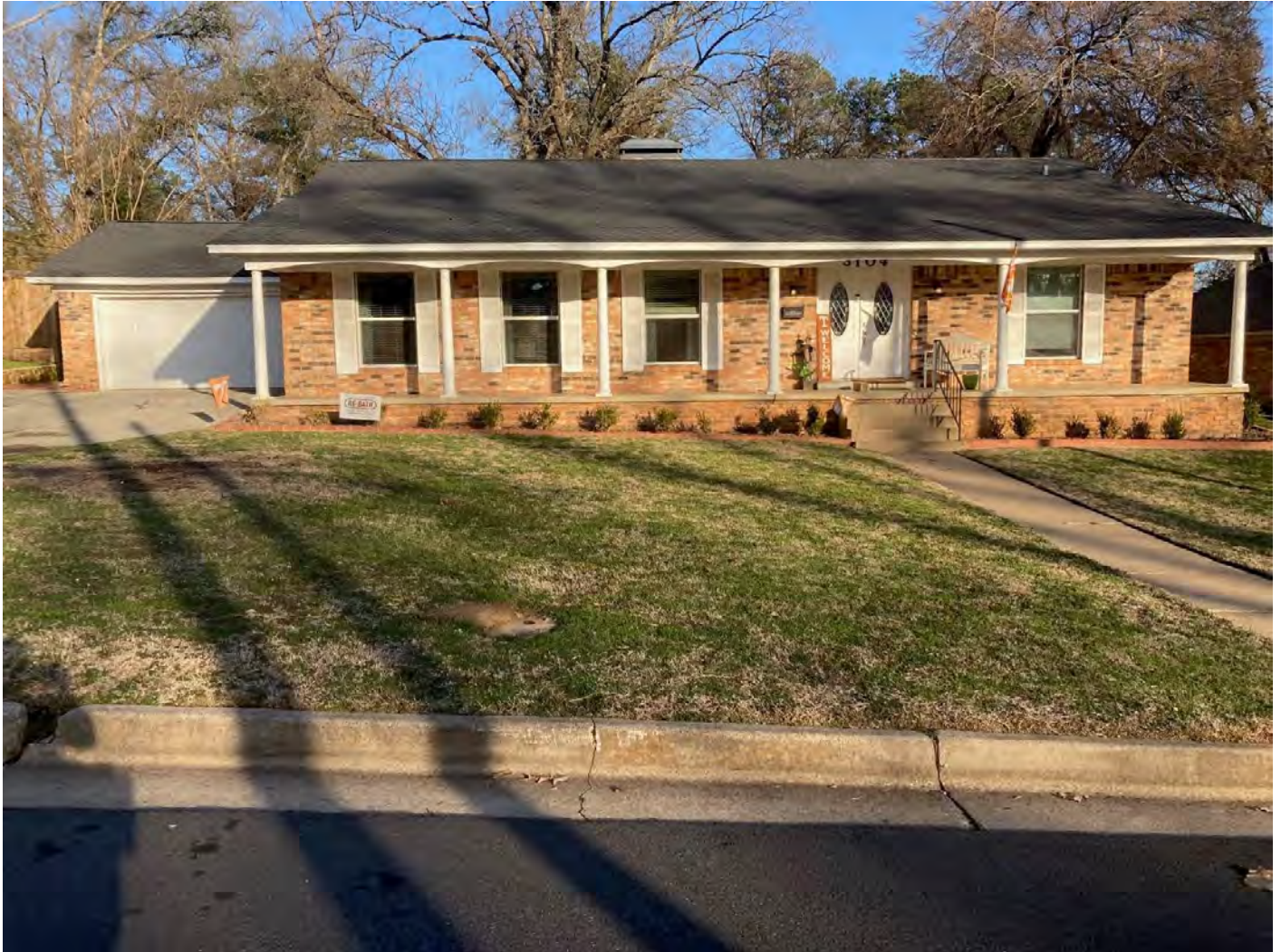
Photo 42. Front façade of 3104 S. Cameron Avenue (Resource 135814). Camera facing southwest.
