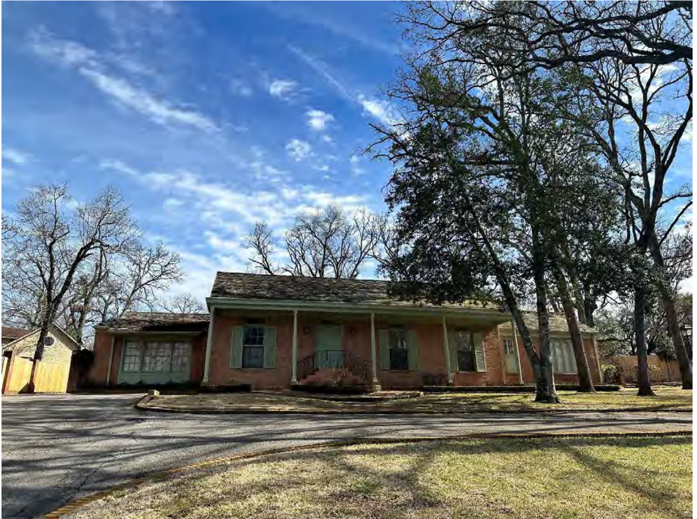
Photo 39. Front façade 2816 Fry Avenue (Resource 138262). Camera facing east.
