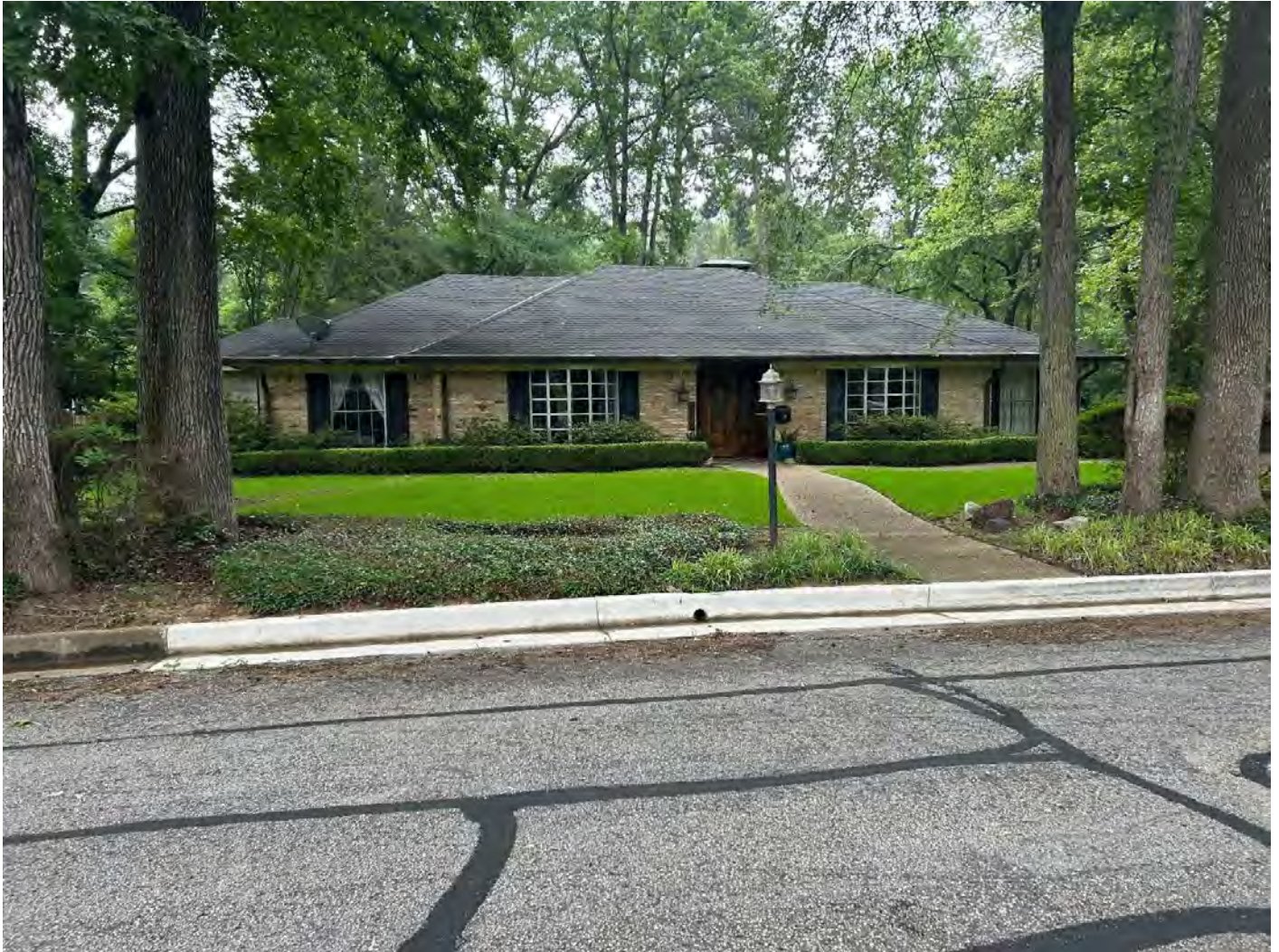
Photo 47. Front façade of 815 Shepherd Lane (Resource 138947). Camera facing southeast.
