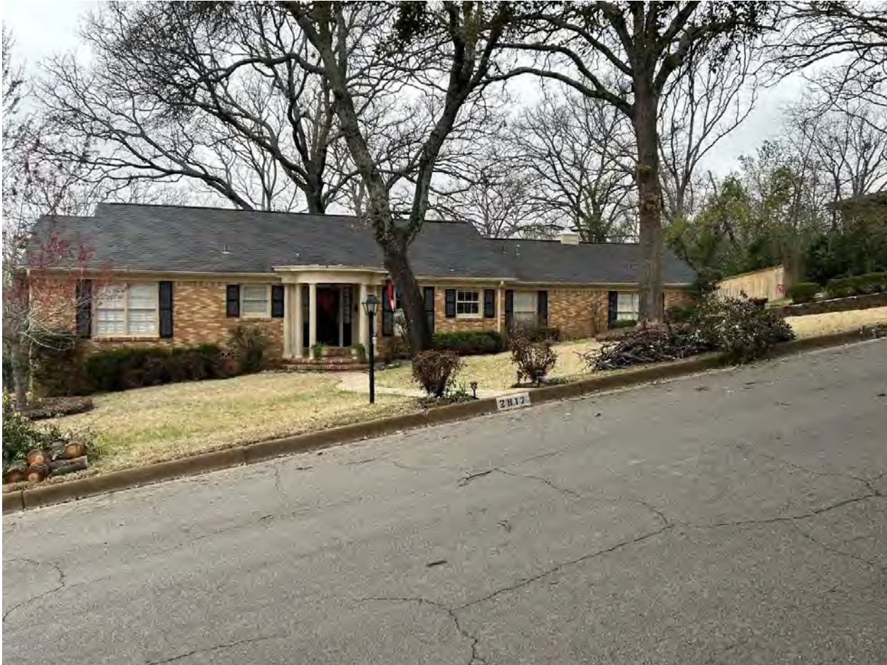
Photo 34. Oblique view of 2917 Curtis Drive (Resource 136086). Camera facing northwest.
