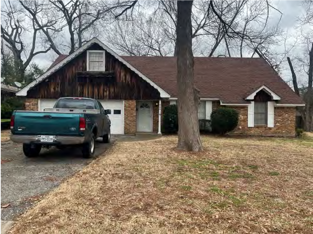
Photo 50. Front facade of 3300 S. Keaton Avenue (Resource 137161). Camera facing east.
