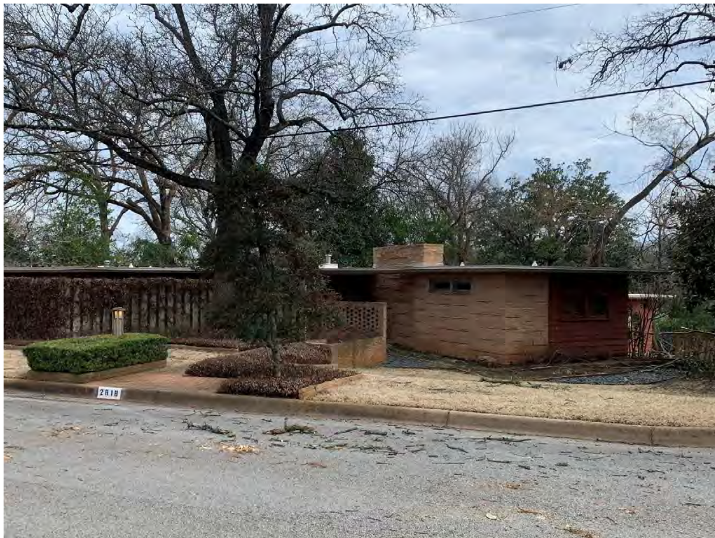
Photo 65. Oblique of 2818 Pounds Avenue (Resource 138297). Camera facing east.
