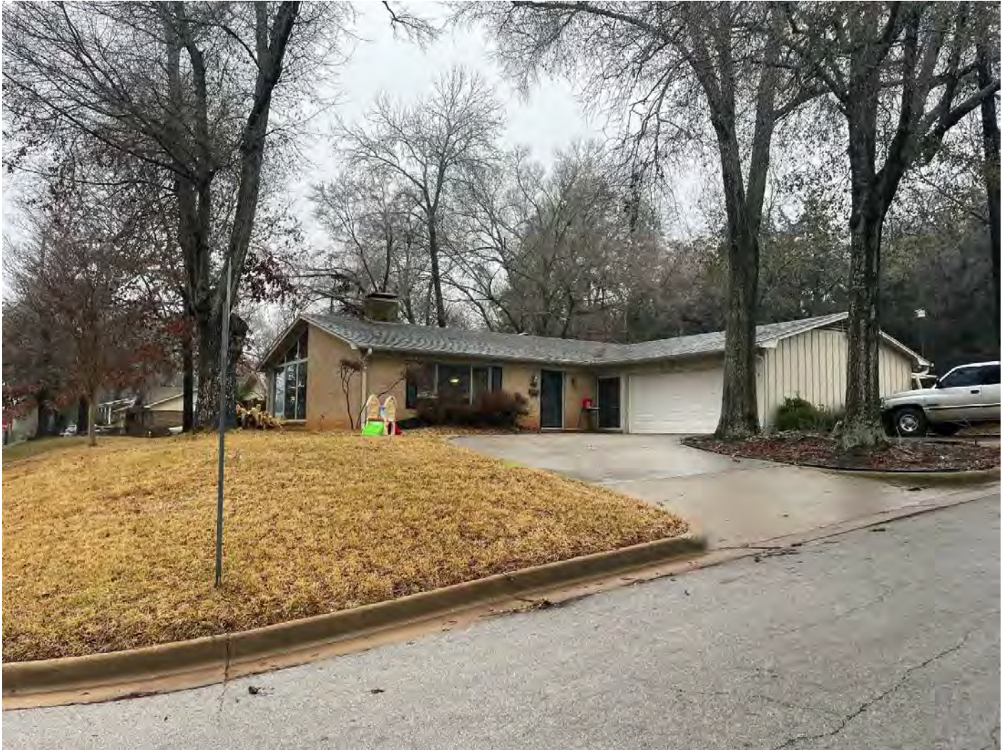
Photo 56. Oblique of 1024 Clyde Drive (Resource 138448). Camera facing northwest.
