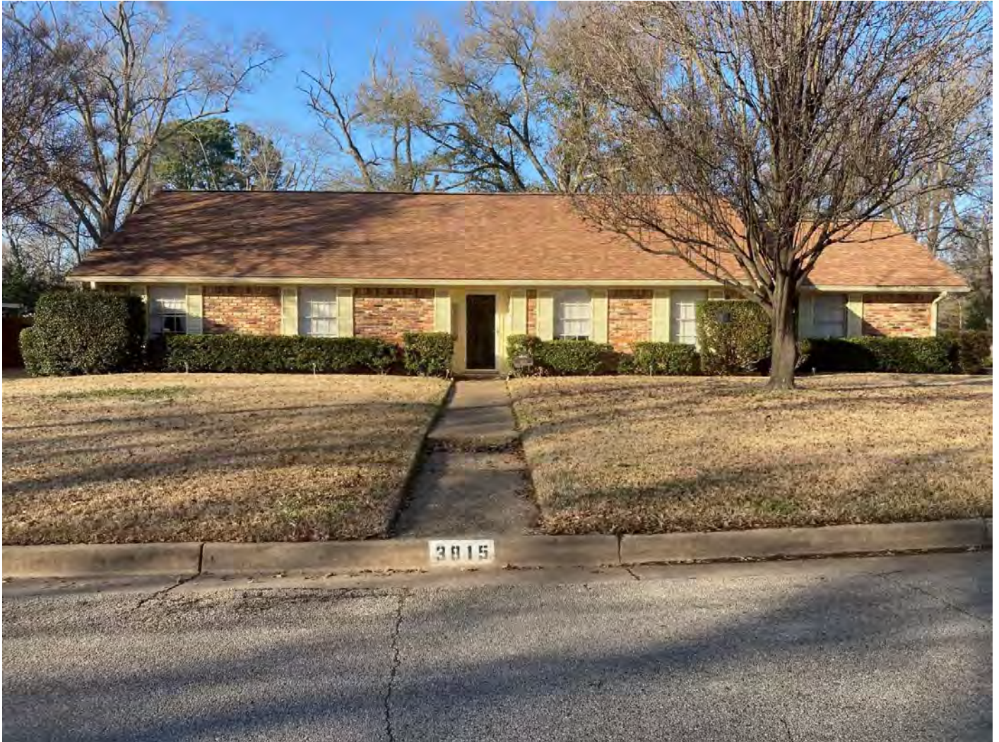
Photo 33. Front façade of 3815 S. Cameron Avenue A (Resource 136521). Camera facing north.
