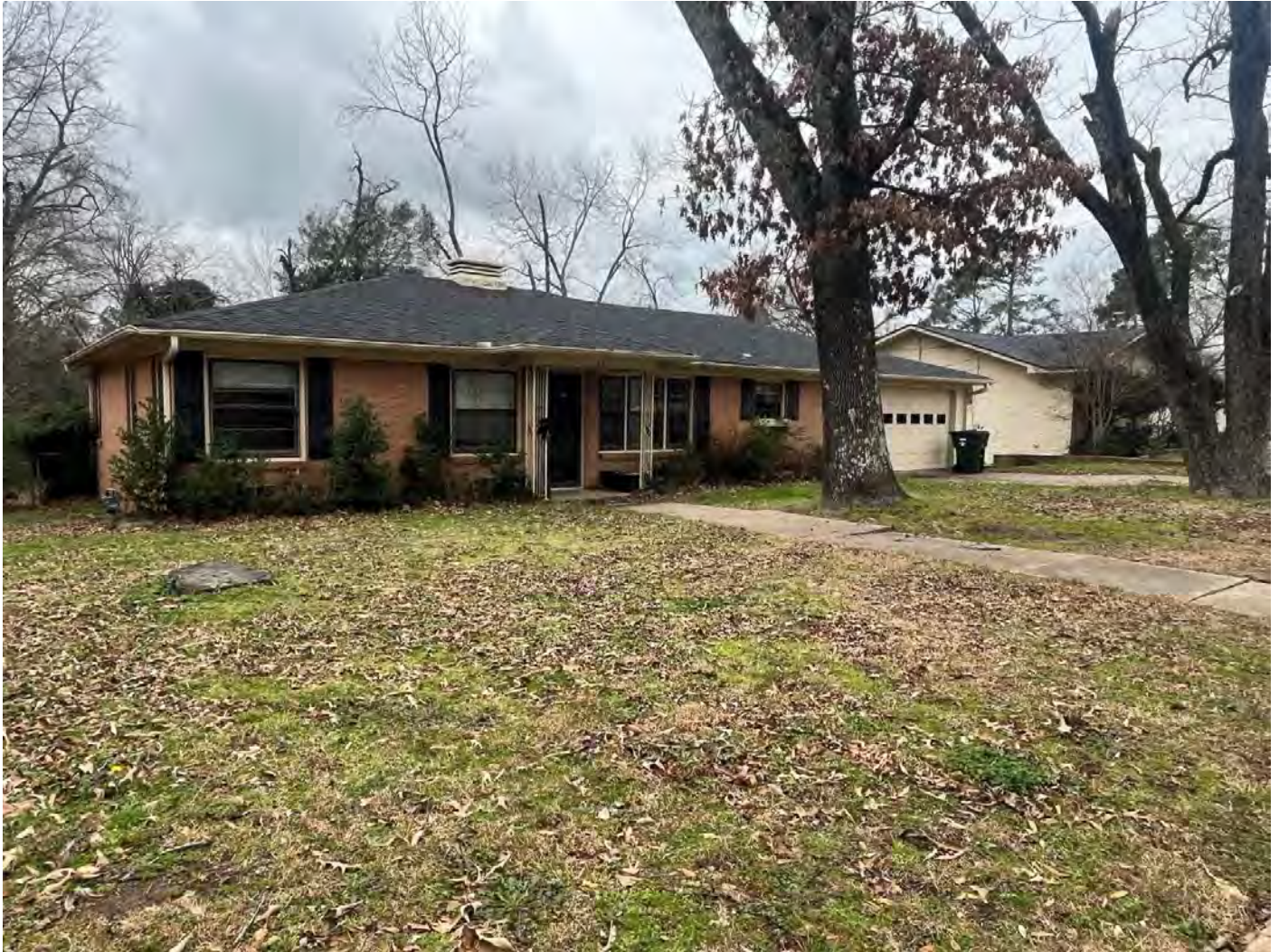
Photo 31. Oblique of 923 E. Hudson Street (Resource 134932). Camera facing southwest.
