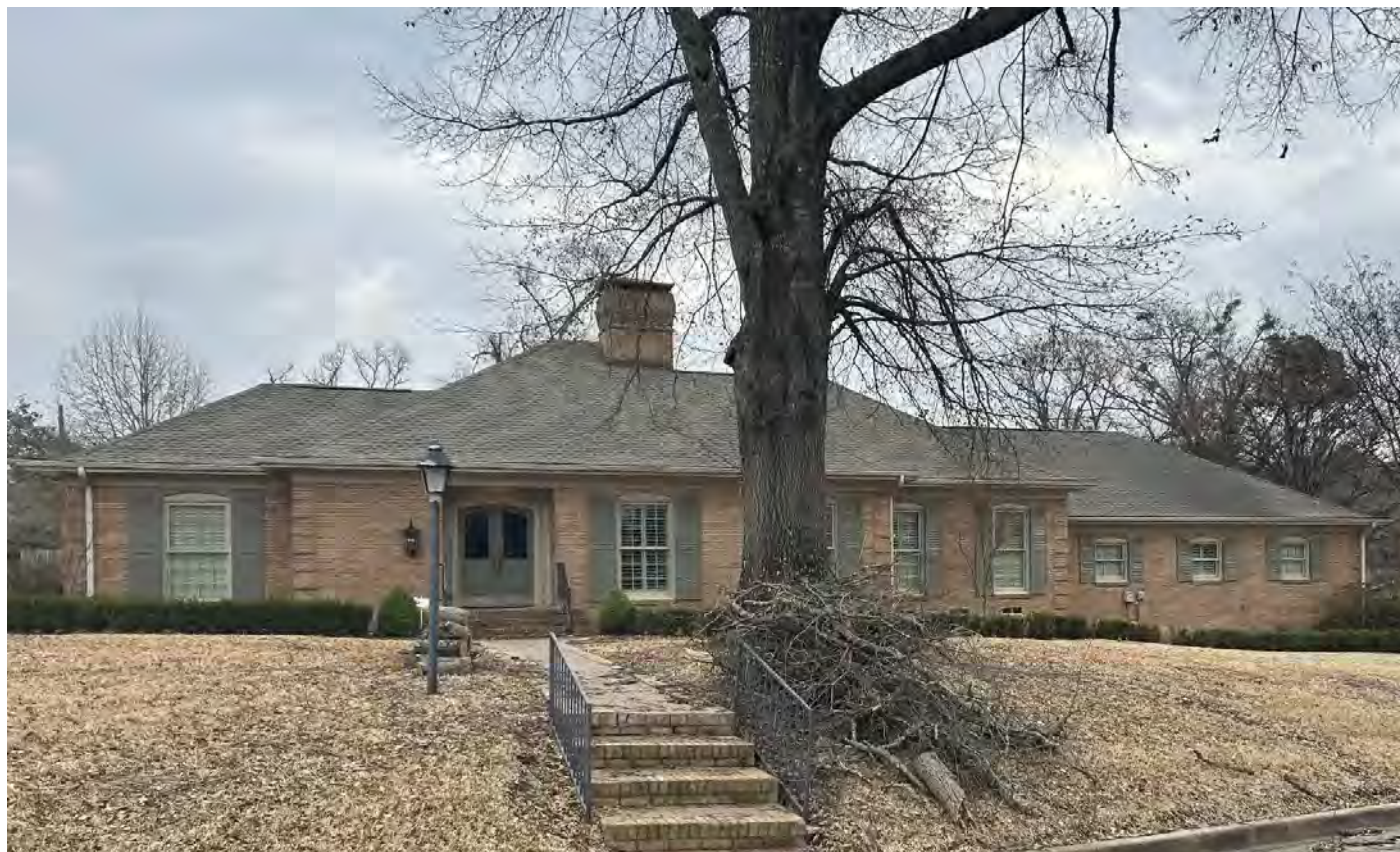
Photo 45. Front façade of 3618 Wynwood Drive A (Resource 138908). Camera facing southeast.
