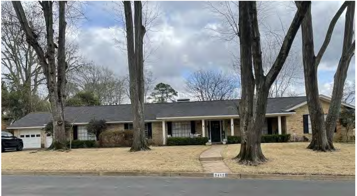
Photo 32. Front façade of 3412 Pollard Drive (Resource 137040). Camera facing east.
