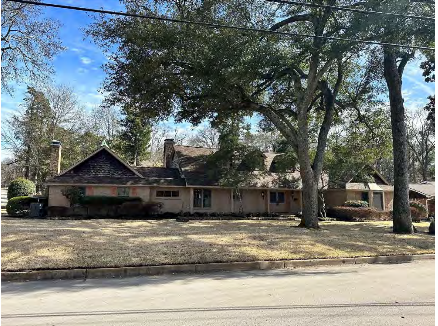
Photo 66. Front façade of 3316 Fry Avenue (Resource 138141). Camera facing east.
