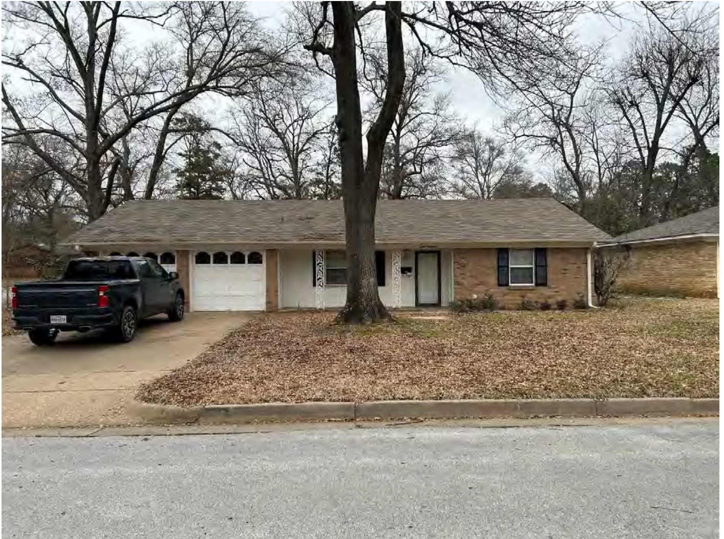
Photo 7. Front façade of 800 Rhodes Drive (Resource 135107). Camera facing north.
