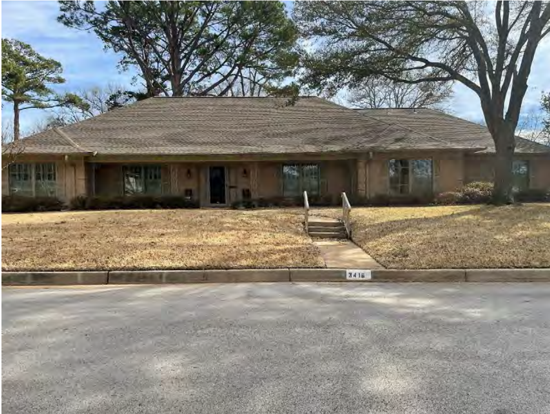
Photo 46. Front façade of 3416 Allen Avenue (Resource 138718). Camera facing east.
