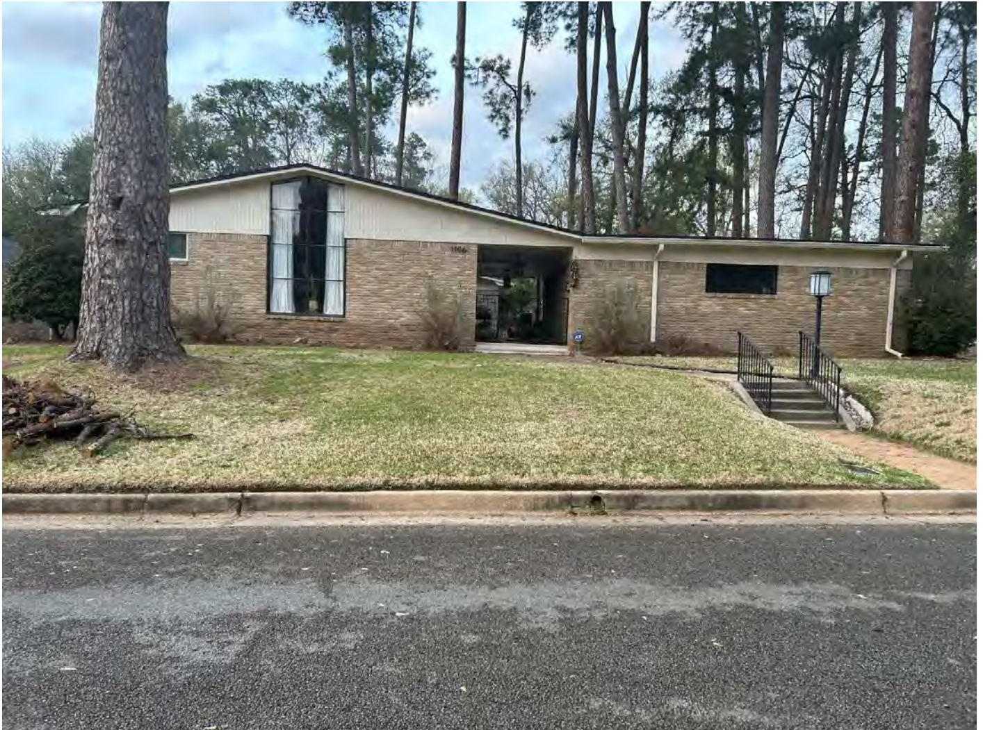
Photo 8. Front façade of 1106 Hansford Place (Resource 138792). Camera facing north.
