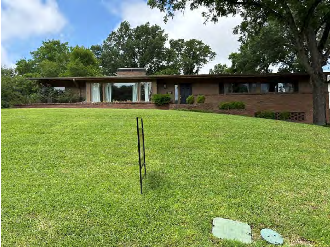
Photo 28. Front façade of 3809 Arlington Avenue (138804). Camera facing southwest.
