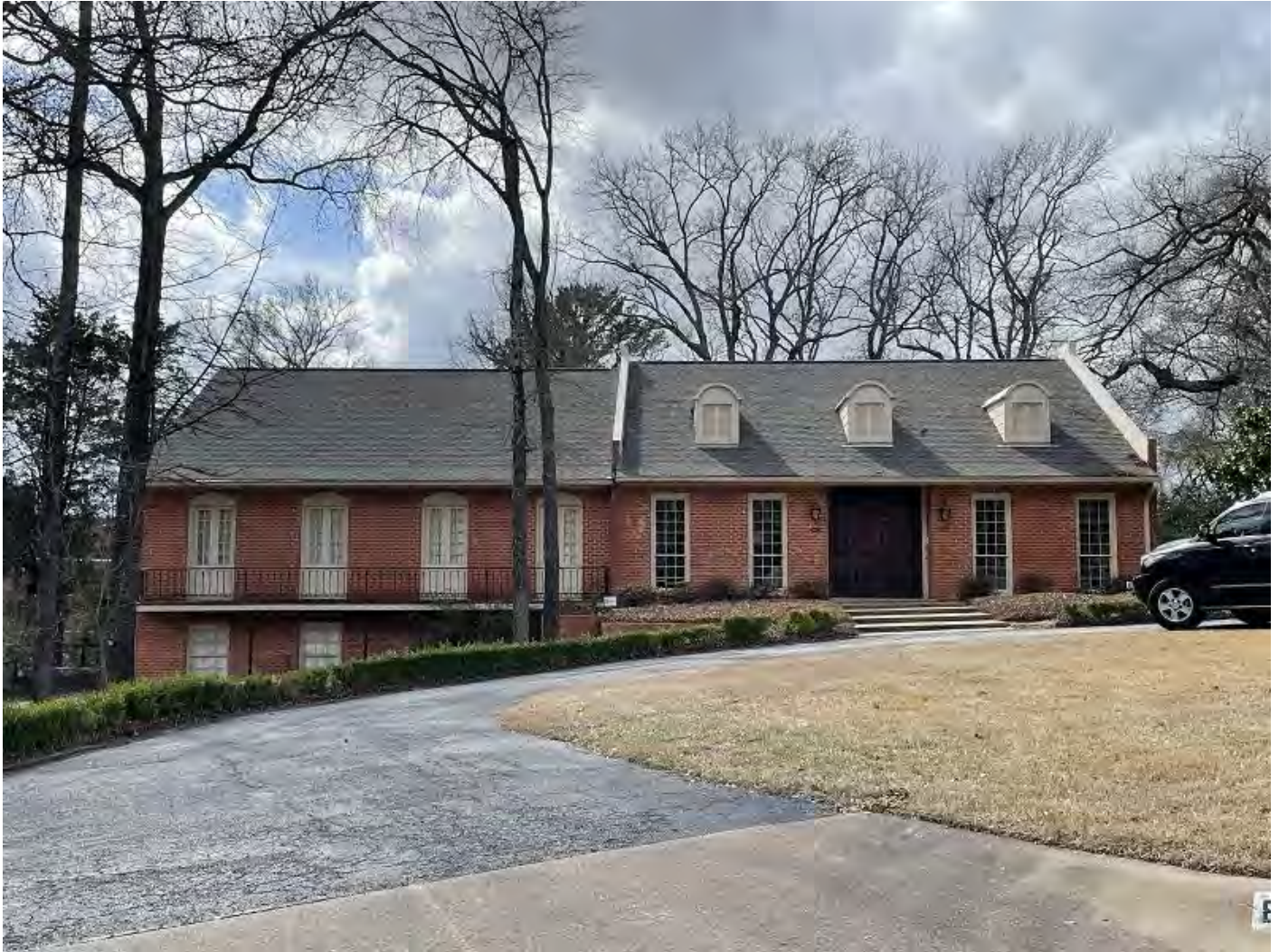
Photo 52. Front façade of 801 Pinedale Place (Resource 139025). Camera facing southwest.
