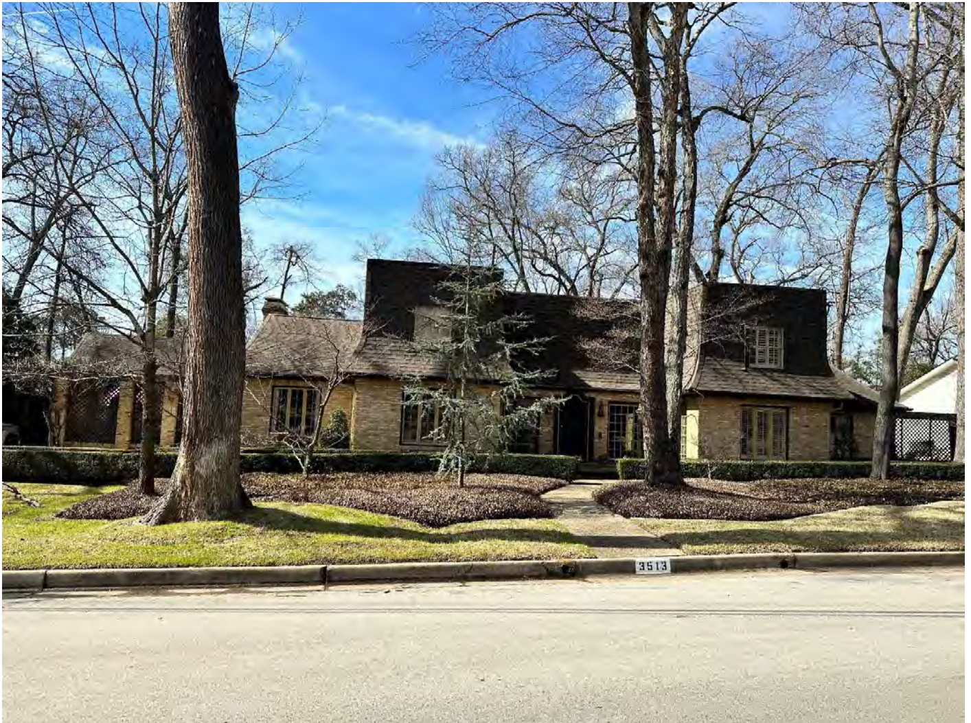
Photo 59. Front façade of 3513 Fry Avenue (Resource 138179). Camera facing west.
