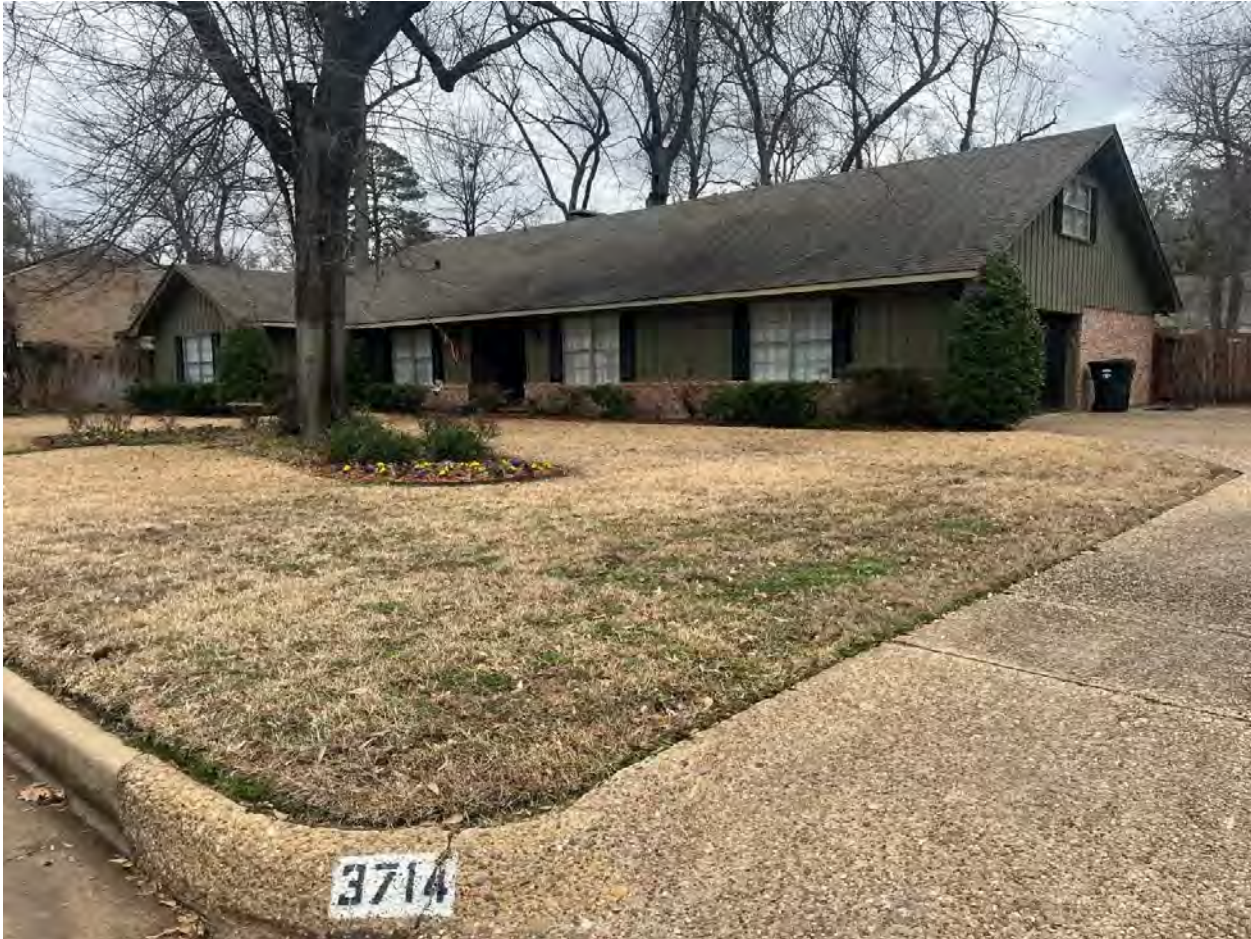
Photo 68. Oblique of 3714 Fry Avenue (Resource 138188). Camera facing northeast.
