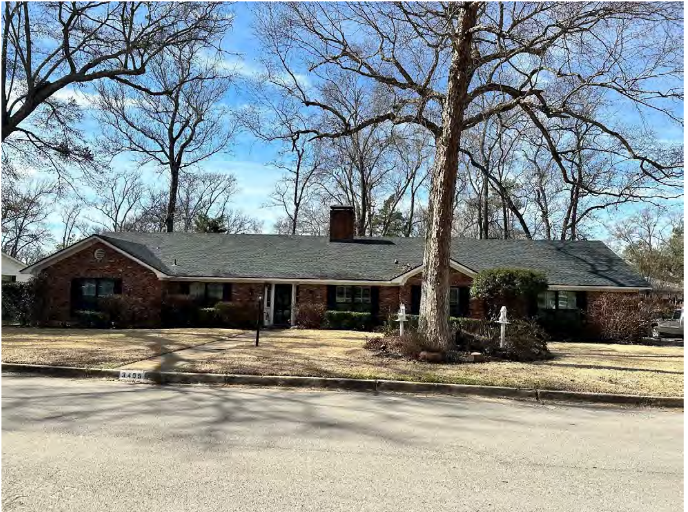
Photo 36. Front façade of 3405 Fry Avenue (Resource 138155). Camera facing west.
