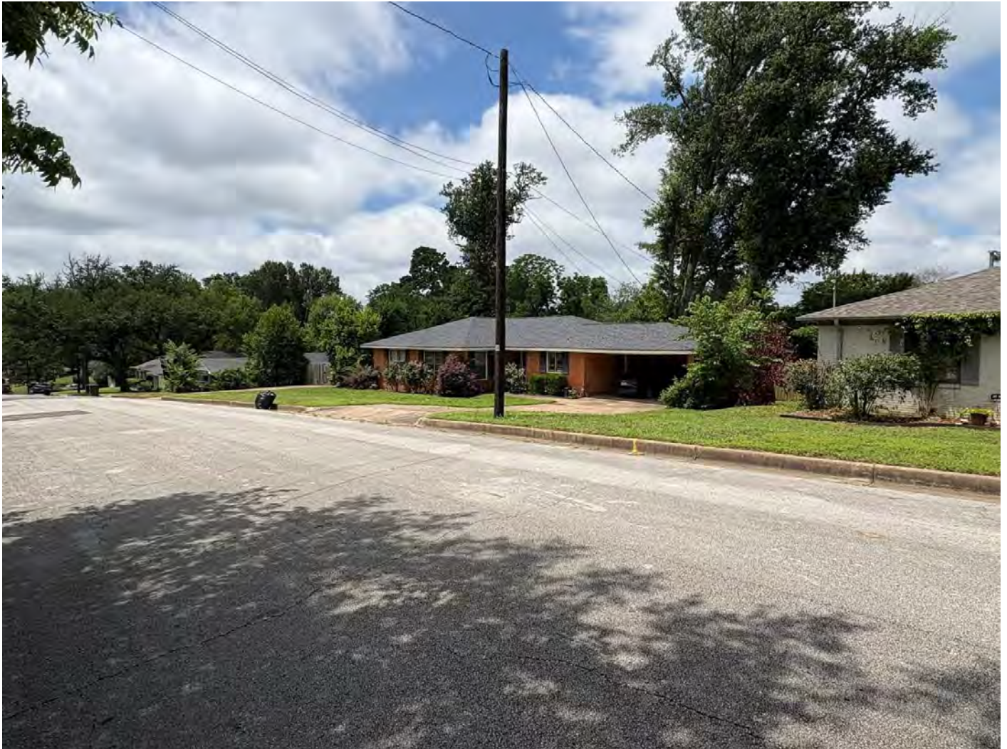
Photo 3. Contextual view of the west side of the 3100 block of Curtis Drive. Camera facing southwest.
