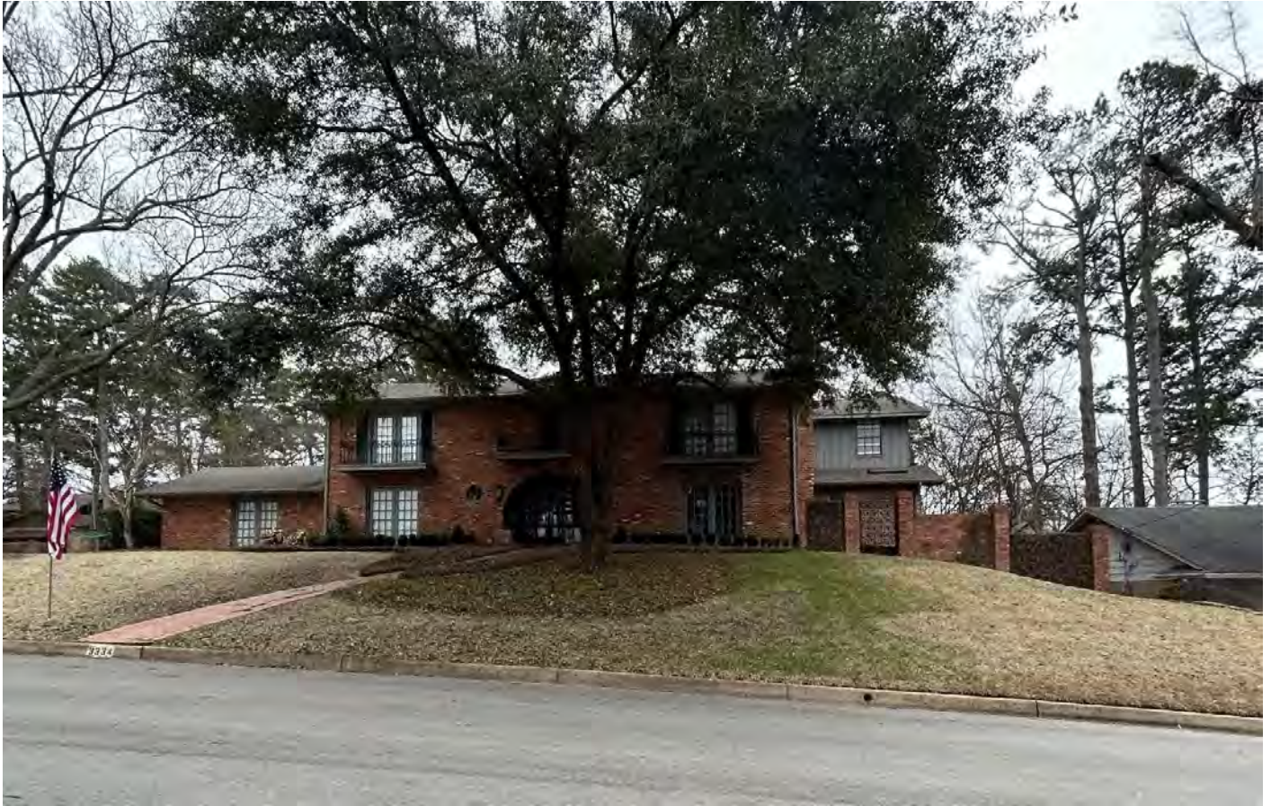
Photo 49. Front façade of 3334 Allen Avenue (Resource 138699). Camera facing east.
