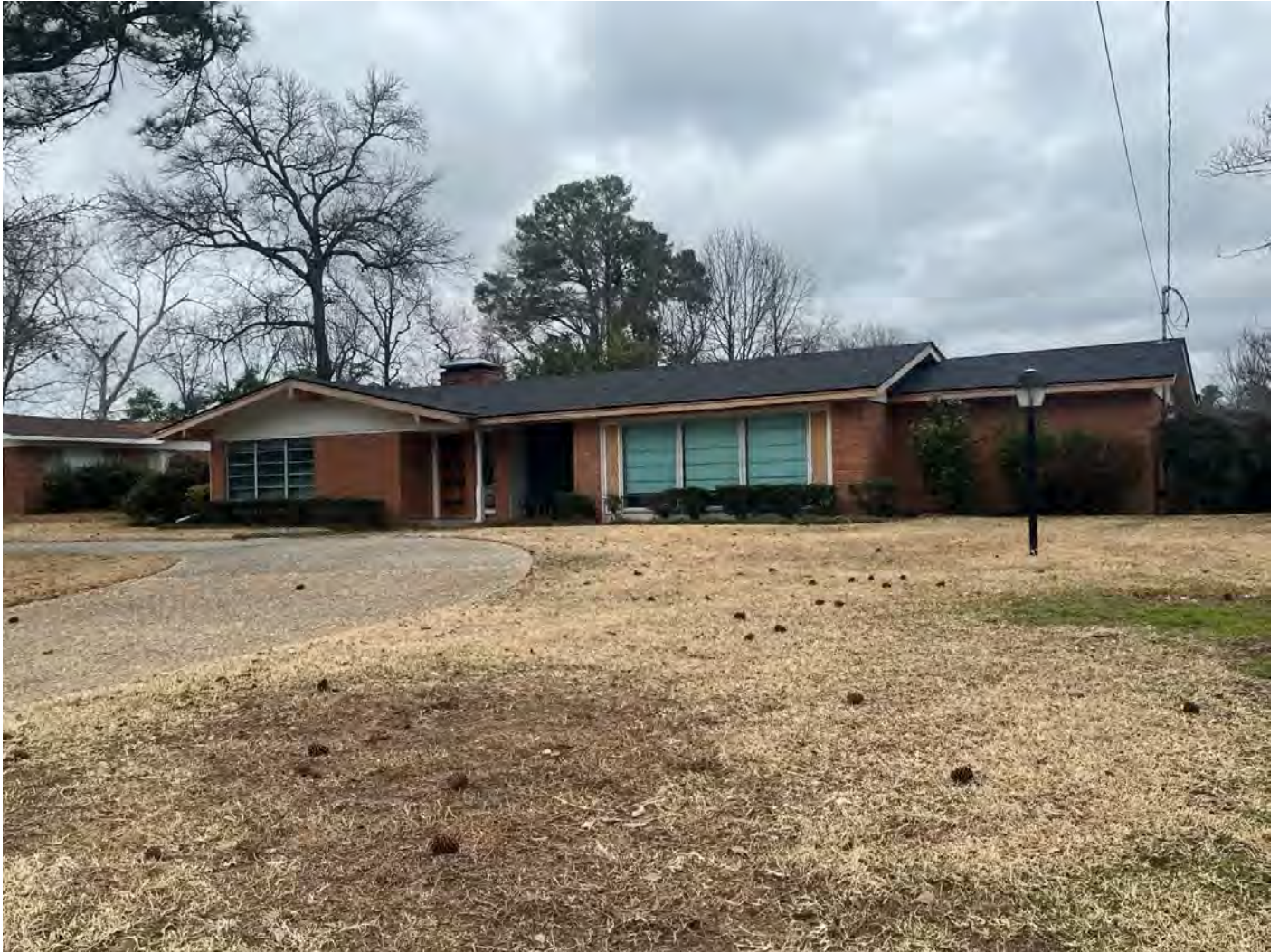
Photo 53. Oblique of 730 Shannon Drive A (Resource 139818). Camera facing northwest.
