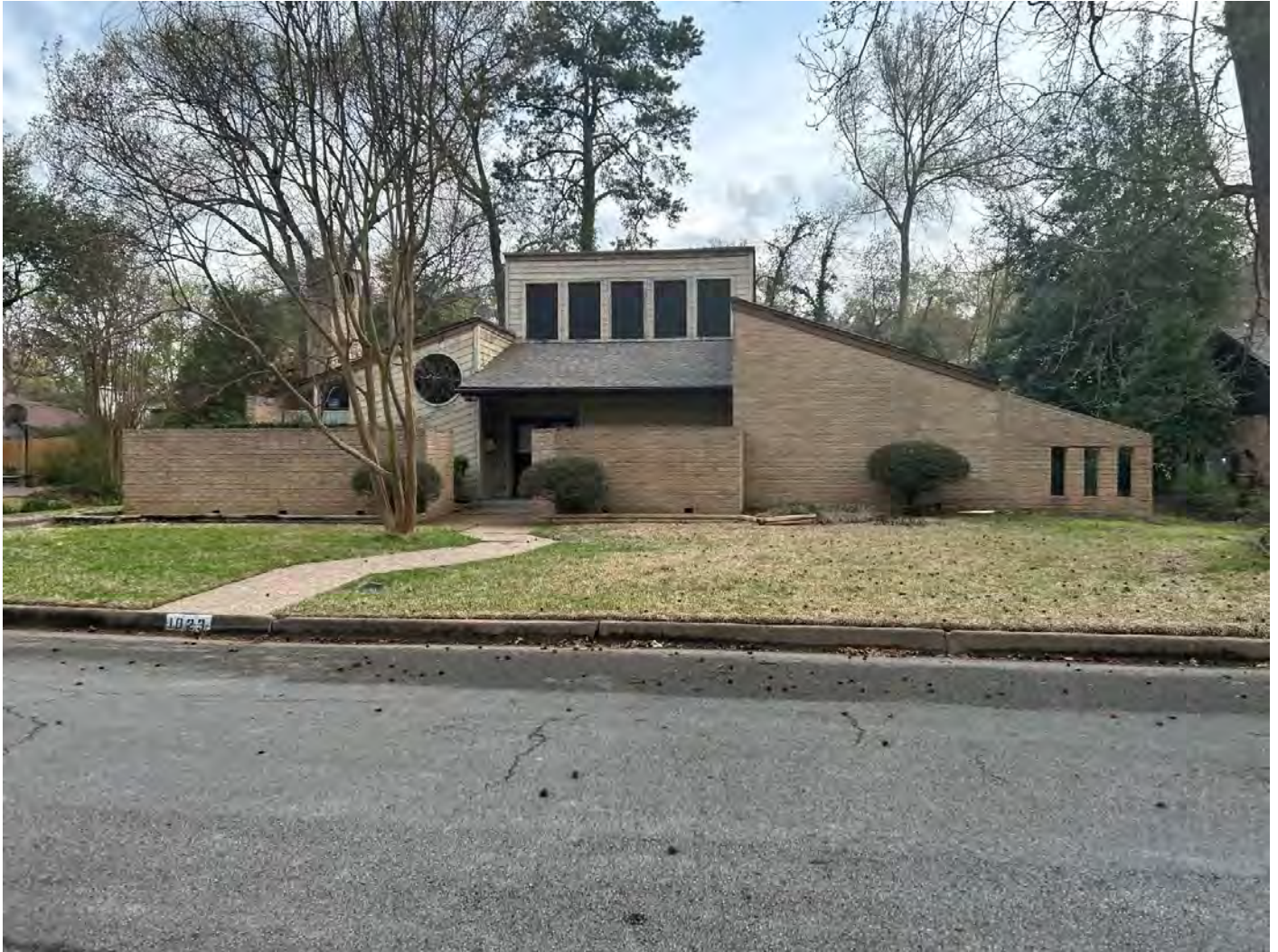
Photo 61. Front façade of 1023 Hansford Place (Resource 139698). Camera facing south.
