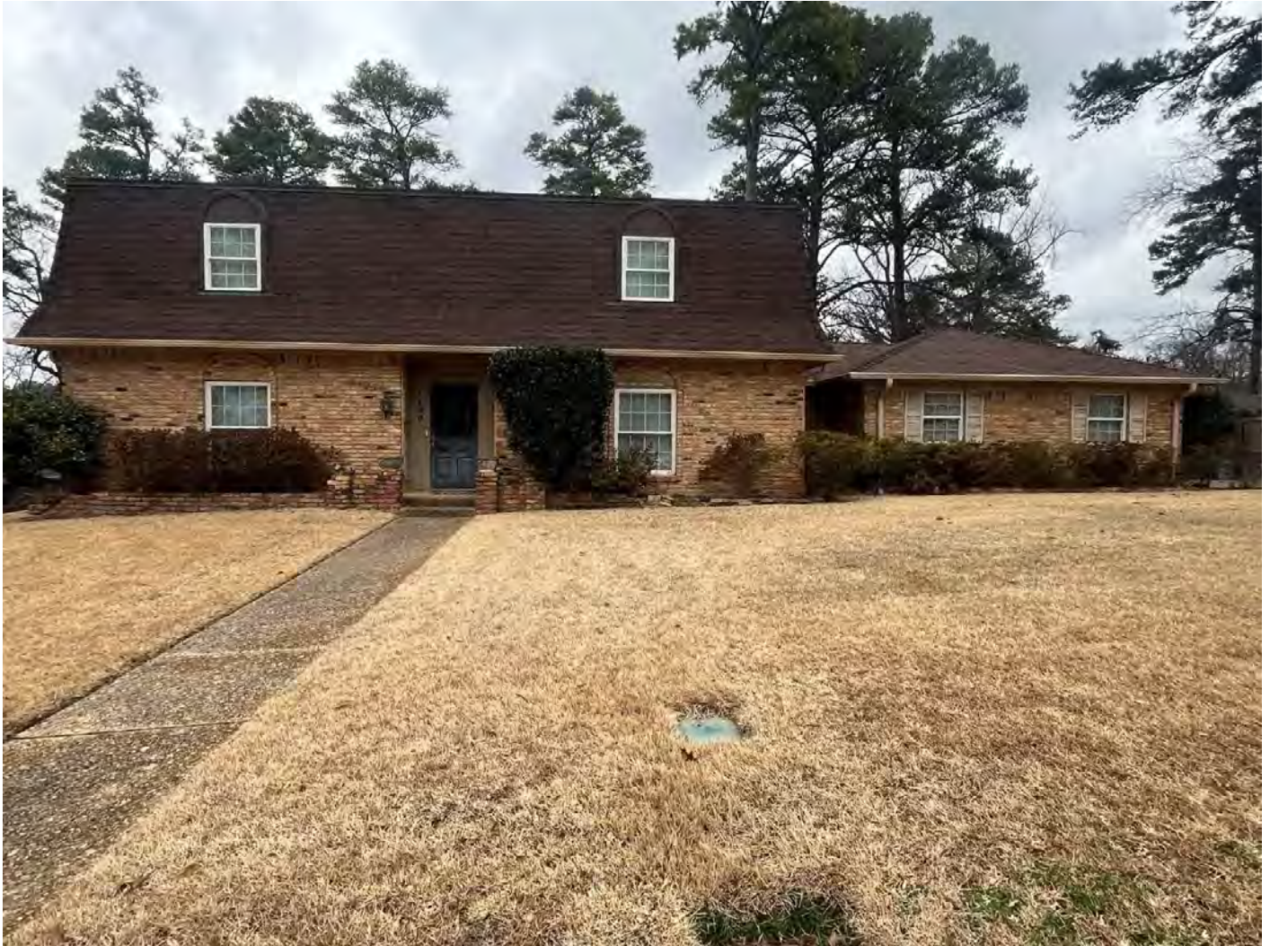
Photo 60. Front façade of 1106 Heines Drive (Resource 138672). Camera facing north.
