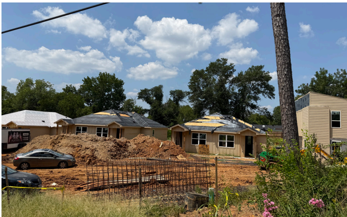
New residential construction showcases the ongoing neighborhood development.
