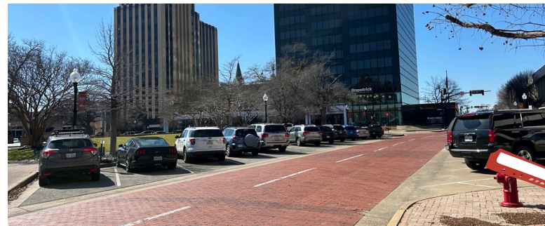
Urban Core Ferguson Street (Collector)
