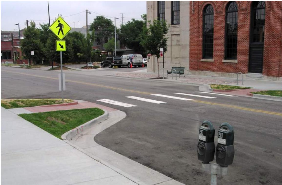
Chokers are a midblock curb extension, reducing vehicular speeds as they navigate through the reduced roadway width.
