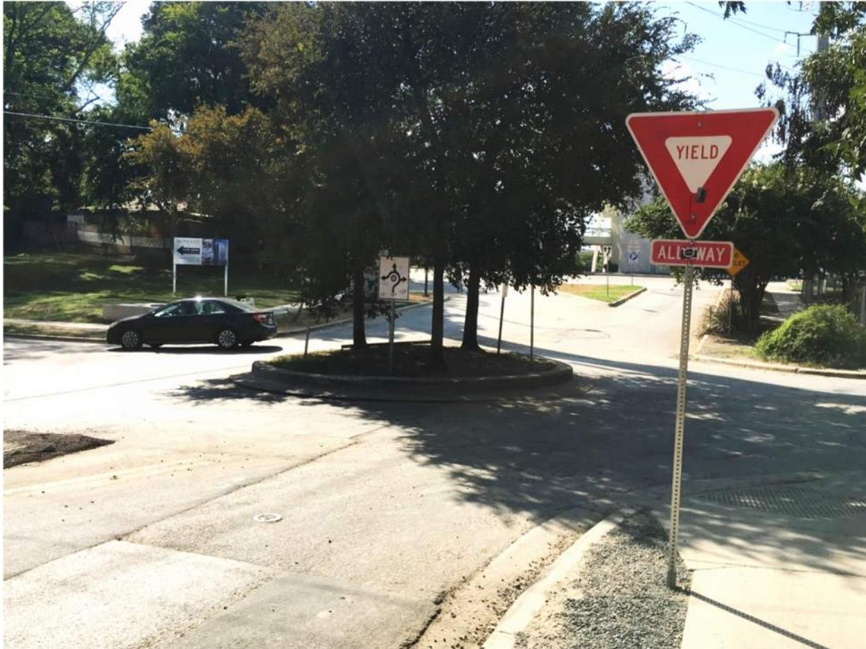
Traffic circles are raised, circular islands at the center of an intersection that force circular movements through the intersection, reducing vehicular speeds.
