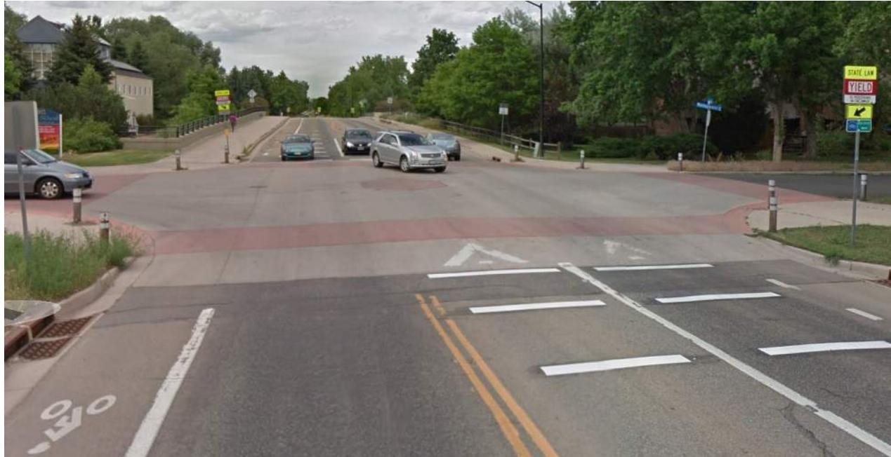
Raised intersections form plateaus that raise intersections to sidewalk height. Ramps leading to the intersection reduce vehicular speeds.
