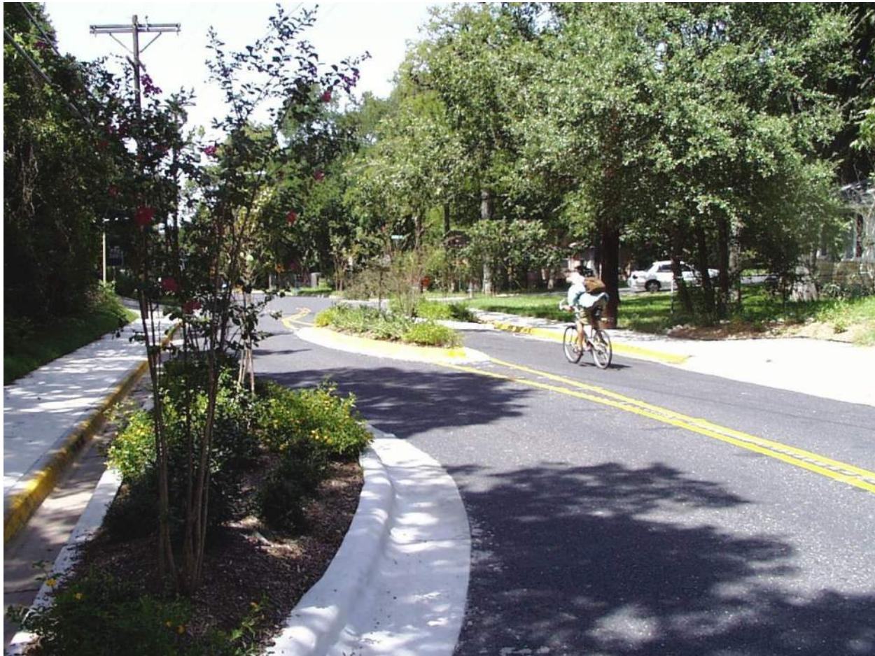
Chicanes provide alternating curb extensions, reducing the roadway width and curving the roadway path, resulting in reduced vehicular speeds.
