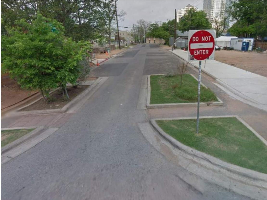
Half roadway closures are created with the placement of a physical barrier to block vehicle traffic in one direction. Pedestrian and bicycle traffic are usually unrestricted.
