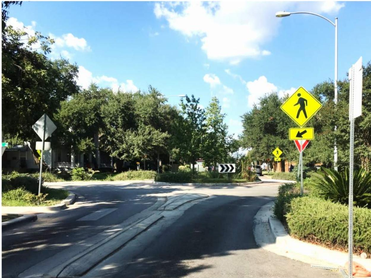
Roundabouts force circular movements at intersections, reducing speeds for navigation and yielding.
