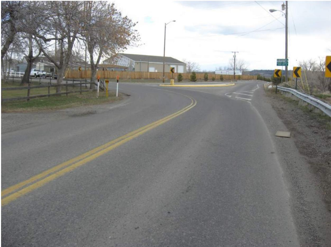
Re-aligned intersections modify existing intersections to add curvature. Previously straight through roadways become curved, slowing down vehicles. Re-alignment is ideal for T-intersections.
