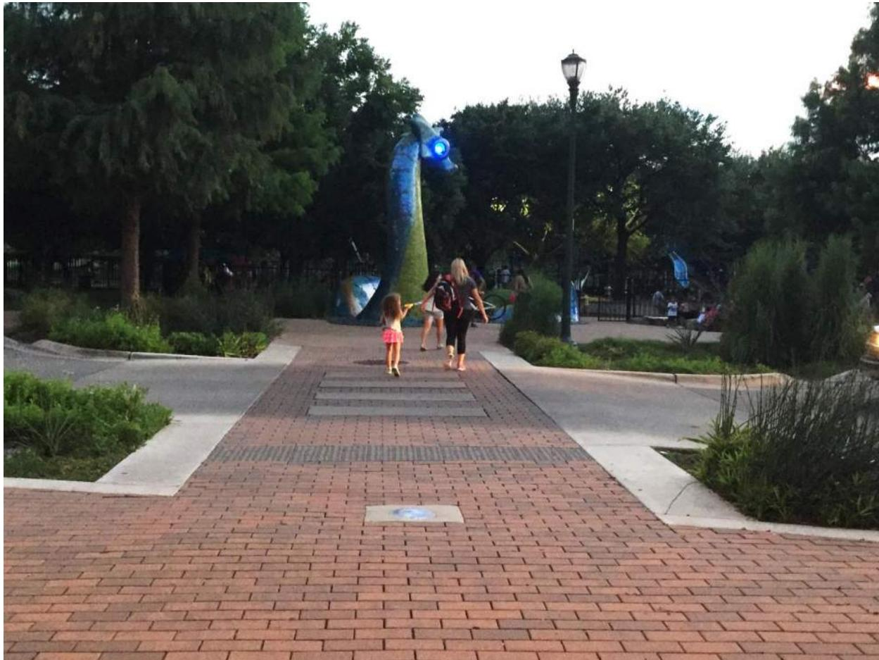
Raised crosswalks are constructed across speed tables coinciding at pedestrian crosswalks. The crosswalks are raised, reducing vehicular speeds and increasing pedestrian visibility.
