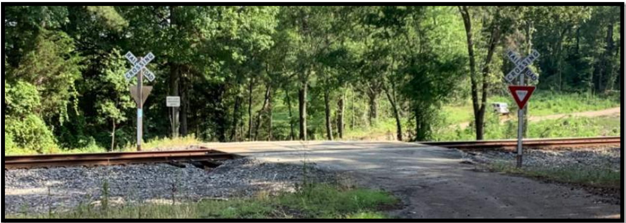
Figure 11: Example of Passive Grade Crossing (DOT # 426644G– CR 253)
