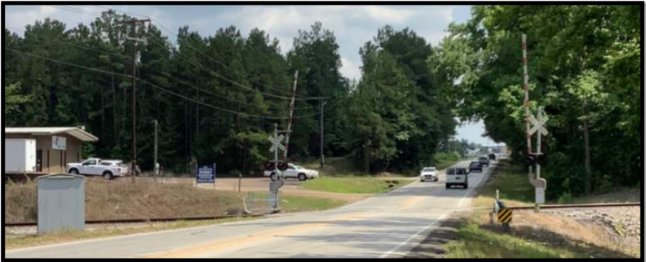
Figure 11: Example of Passive Grade Crossing (DOT # 426644G– CR 253)
